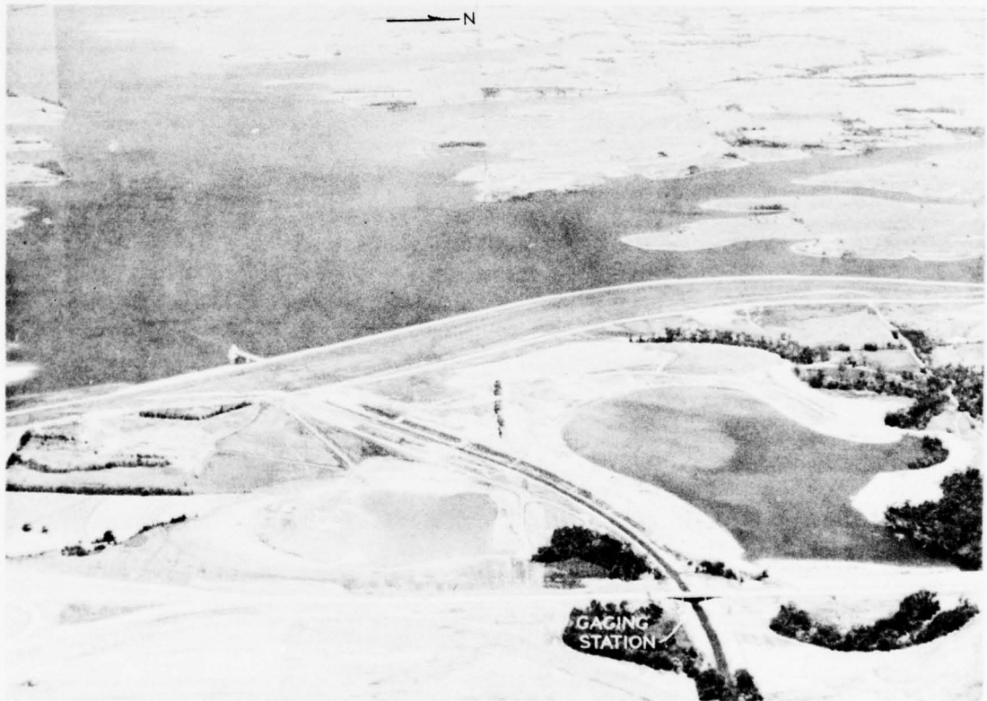
Figure 1. Melvern Dam, Kansas
