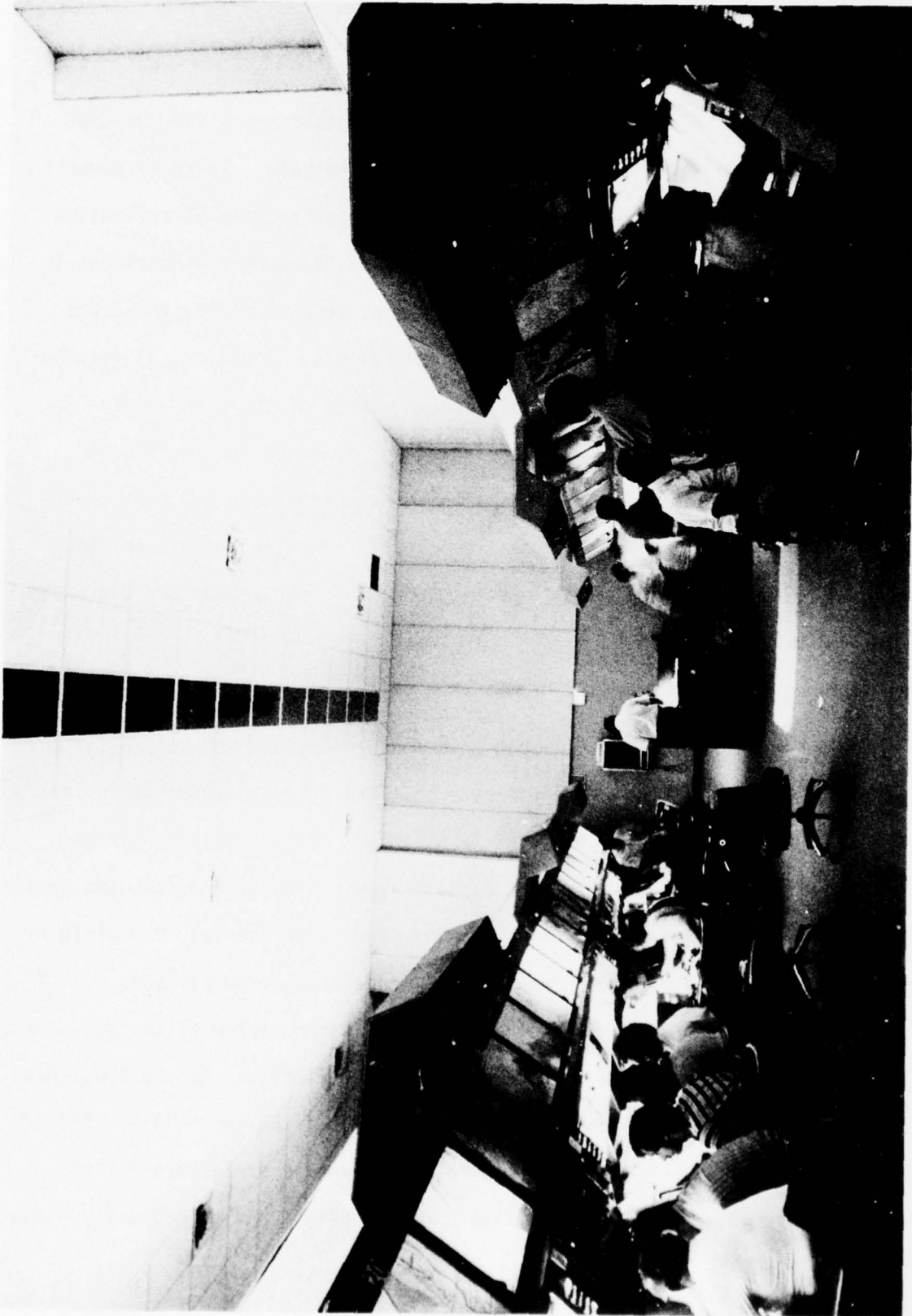
FIGURE 7.1 - BALANCED AMBIENT ILLUMINATION WITH MAP BOARD LIGHTS DIRECTED TOWARD THE AISLE
