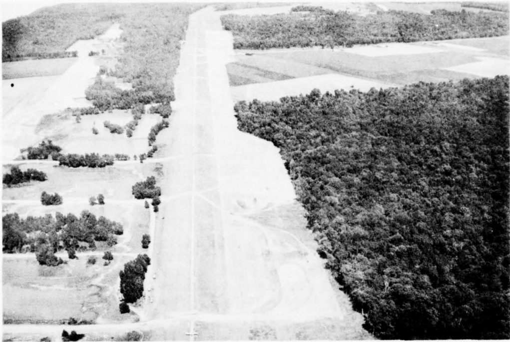
Mississippi River Levee. Landside seepage berm under construction.
