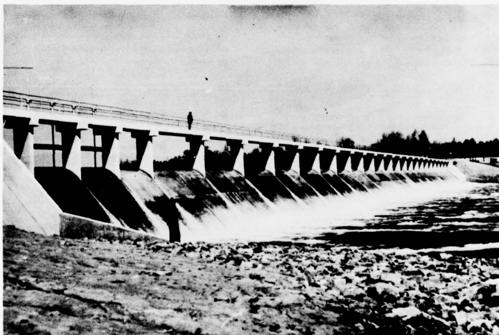
Lake D'Arbonne Spillway, Union Parish, Louisiana.
