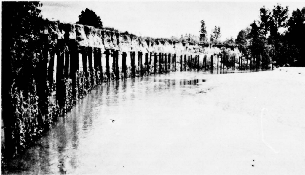
Bank stabilization on Upper Big Sand Creek, Yazoo River Watershed Project.
