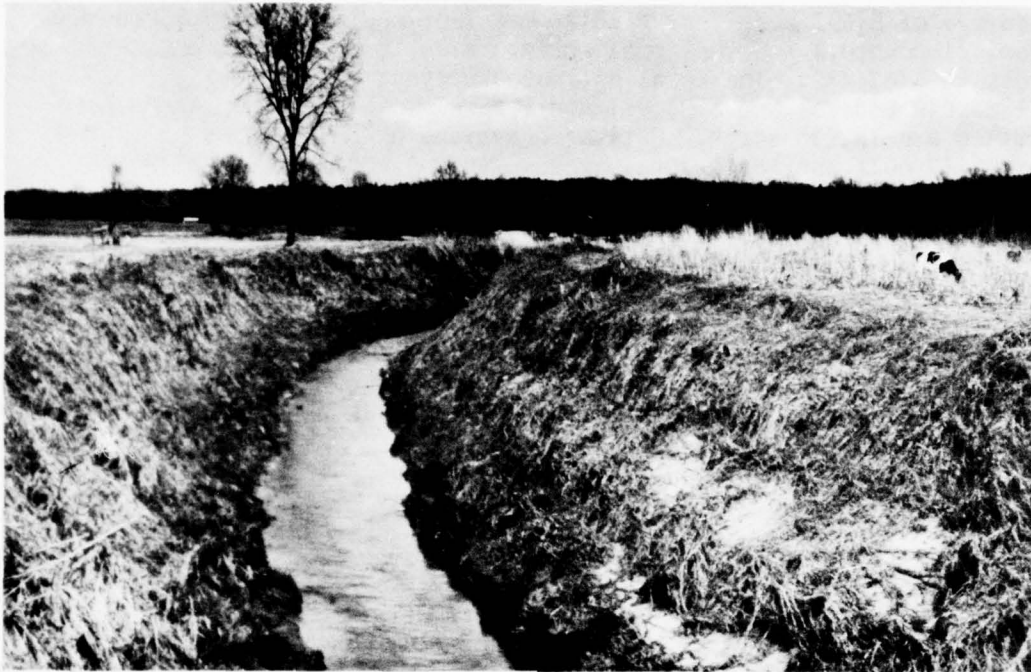
Typical watershed project - Kudzu keeps down willow growth and protects banks. Adequate drainage and flood protection increase land productivity.
