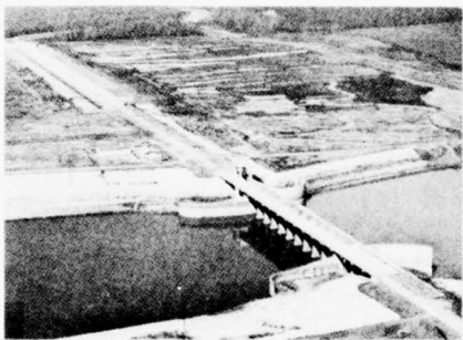
Old River control structures
