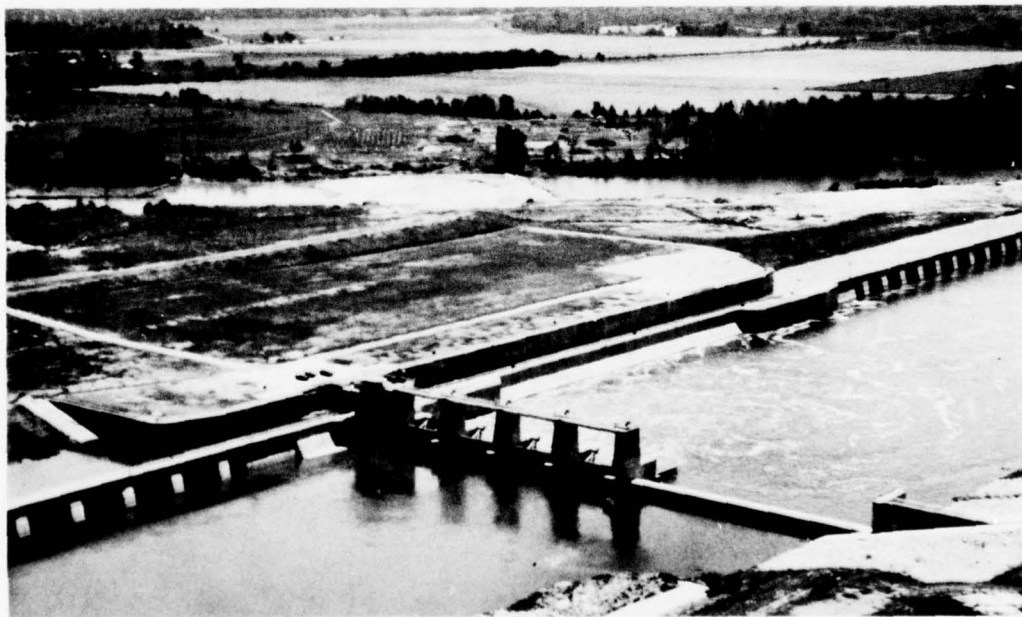
Columbia Lock and Dam, Columbia, Louisiana.
