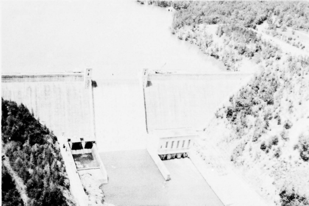
Aerial view of Narrows Dam and Lake Greeson on Little Missouri River.
