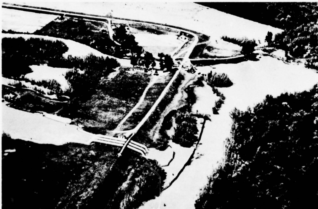
Marked Tree Siphon, Marked Tree, Arkansas, in operation, St. Francis River.
