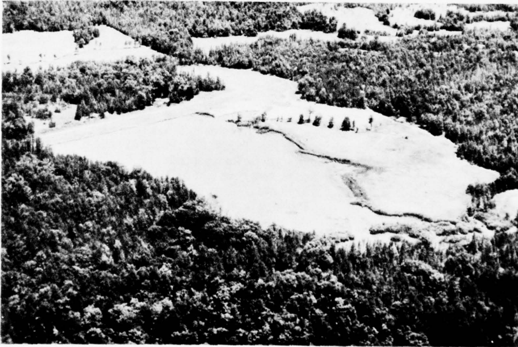
Aerial view of floodwater retarding structure on typical watershed project.
