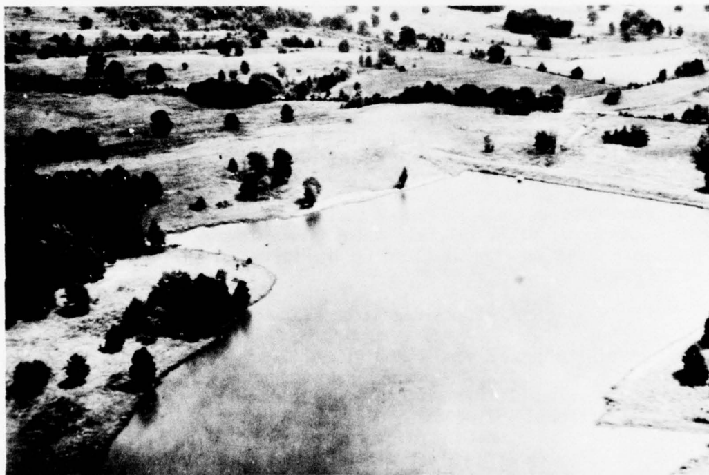
Typical floodwater retarding structure.
