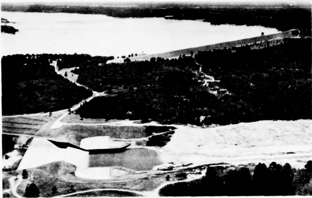
Arkabutla Lake and Dam showing spillway in foreground and dam and lake in background.
