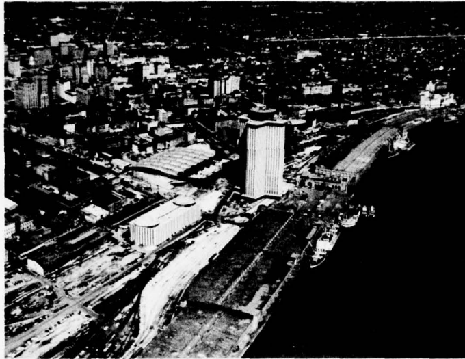
New Orleans, the largest city in the region, endures all the complex problems of congestion in a typical large metropolitan area
