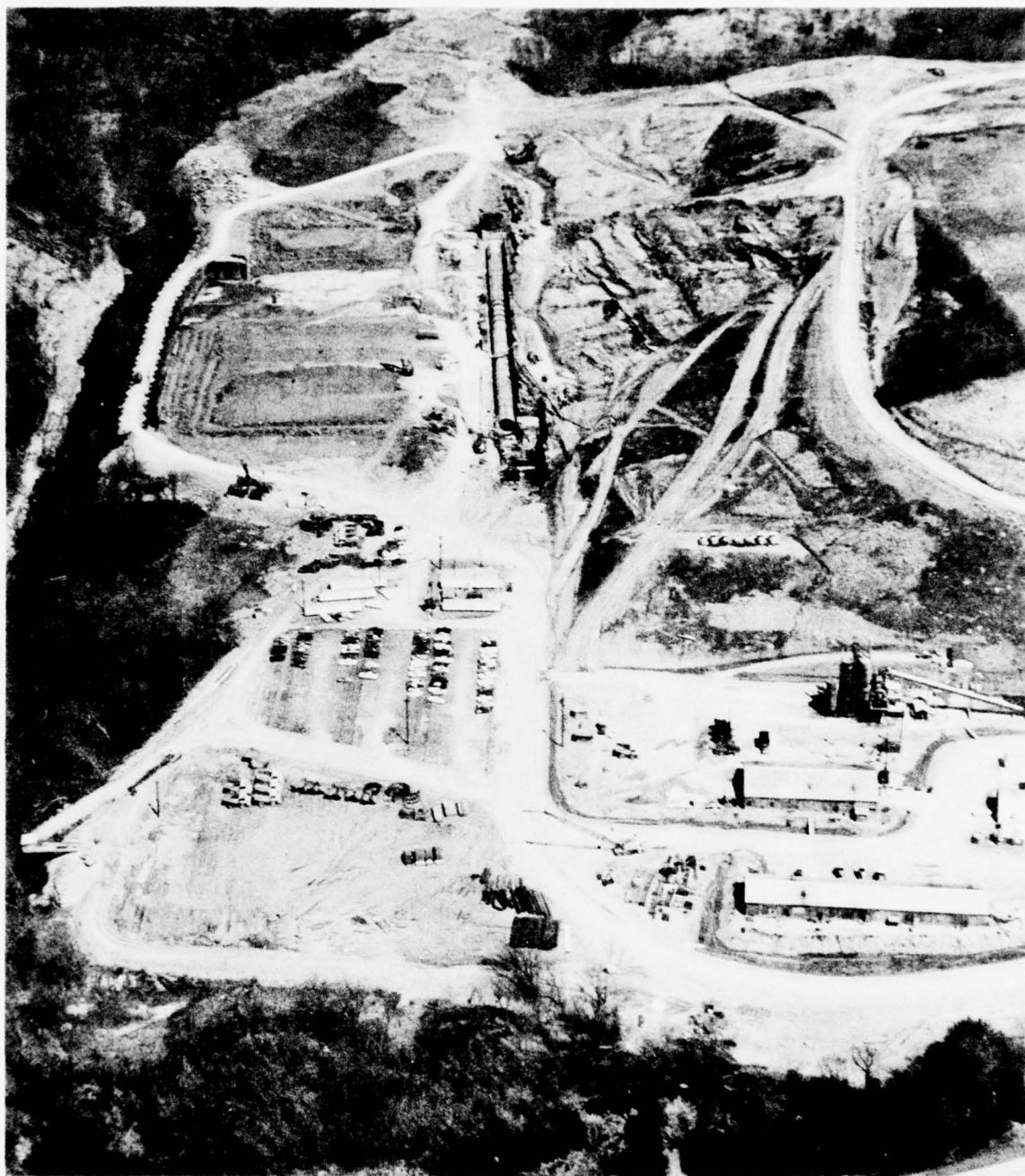
FIGURE 20-12 -- Tims Ford Dam on Elk River in First Construction Stage, March 26, 1968
