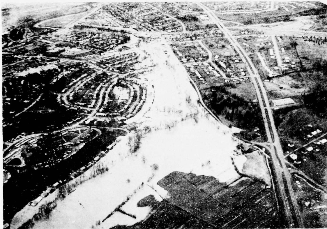
FIGURE 20-2 -- Flood of March 12, 1963 -- Reedy Creek at Kingsport, Tenn.
