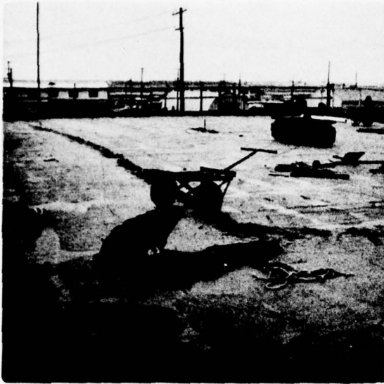
3. Contractor began removal of existing BUR on 6 July 1971.
