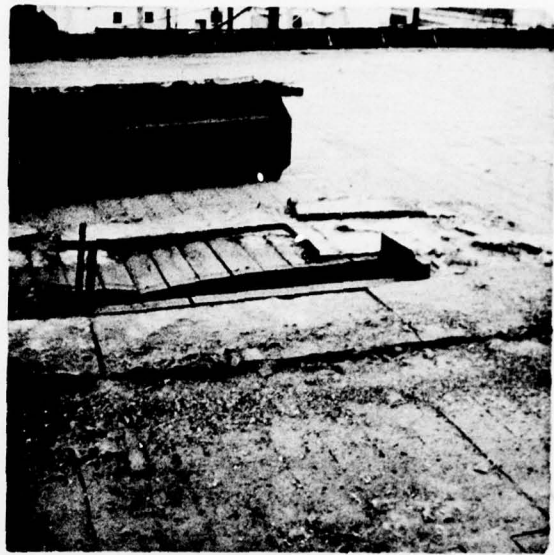
4. Metal deck, insulation and metal deck at ridge vent.
