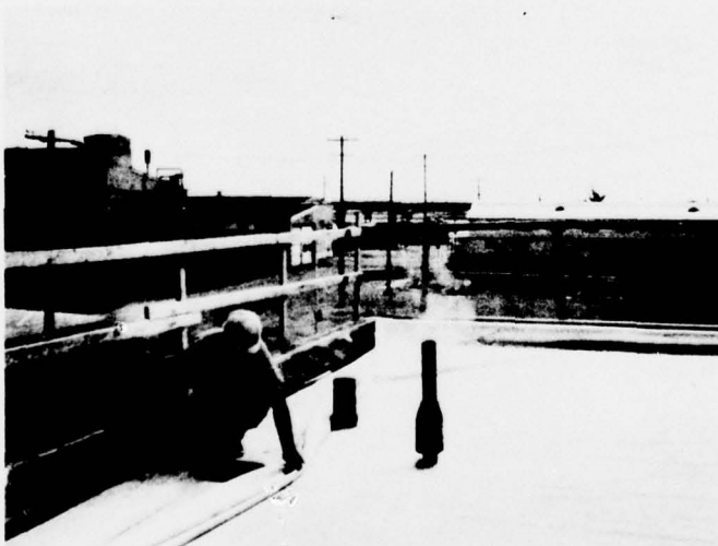
14. Exhaust stack and waste vent penetrations.
