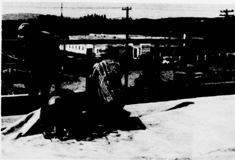
12. Cutting membrane for roof penetrations.
