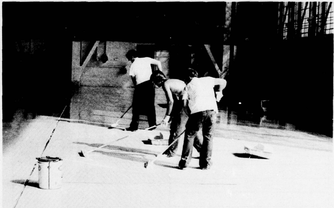
Figure 8. Application of System A with lamb's wool applicators.
