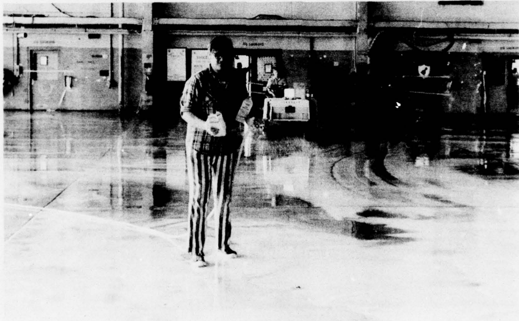
Figure 3. Application of water and industrial grease remover to hangar deck.
