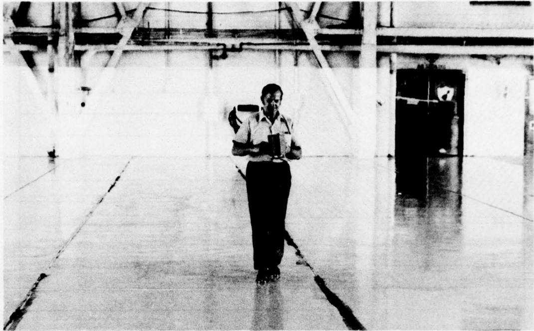
Figure 7. Applicator wearing golf shoes broadcasts grit into first wet finish coat using a grass seeder.
