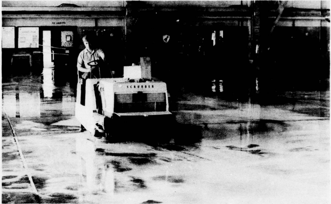
Figure 4. Hangar deck thoroughly scrubbed during the grease removal phase.
