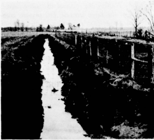
Figure 2.9 Farmland Drainage by Ditching Is a Widely Employed Improvement in the Coastal Plain of the Southeast.
