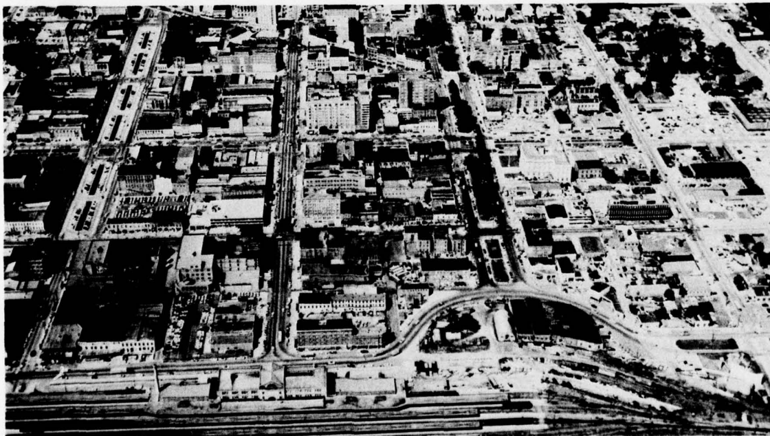
Figure 4.12 Macon—One of Three Metropolitan Cities on the Fall Line in Georgia.
