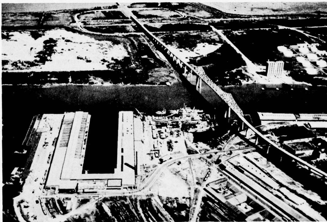
Figure 2.17 Port Facilities — Eugene Talmadge Memorial Bridge, Savannah.
