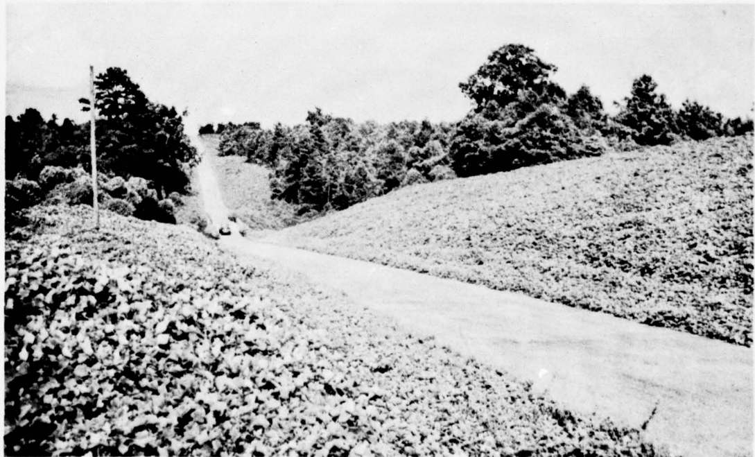
Figure 2.30 Kudzu Protects Roadbanks from Erosion.
