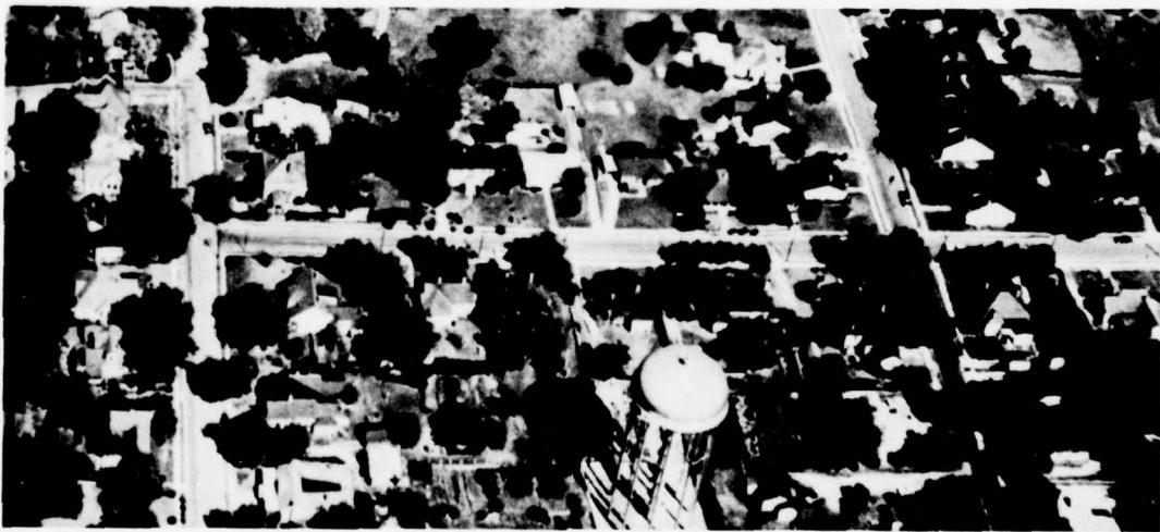
Figure 2.8 Elevated Water Storage Tank — Elberton, Georgia.
