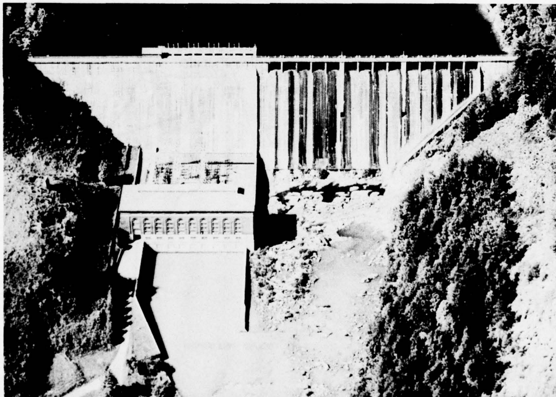
Figure 2.23 Tugaloo Dam and Powerplant — 110 Million Kilowatt-Hours Are Generated Annually.
