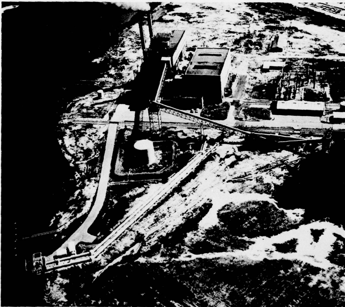
Figure 4.5 Steam Powerplant, near Savannah, Showing Intake and Other Water Supply Facilities.
