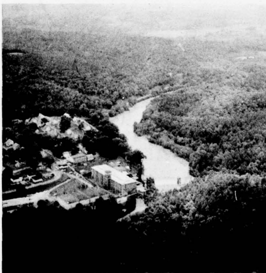
Figure 4.24 Courtenay Powerplant and Mill, Newry, South Carolina, Is Located Just Downstream from the Newry Site.
