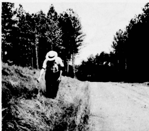
Figure 2.44 Roadside Cuts Stabilized with Love Grass and Bermuda Grass Reduce Sediment Deposition.
