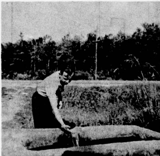
Figure 1.13 Considerable Water Flows from Uncapped Artesian Wells.
