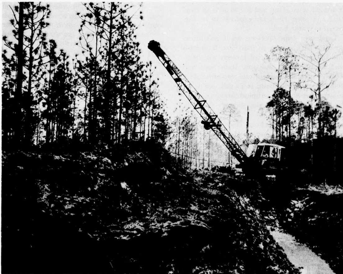
Figure 4.3 Woodland Water Control Project Under Construction.
