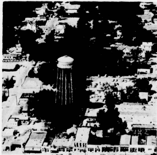
Figure 2.4 Municipal Water Storage Tank, Thomasville, Georgia.
