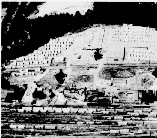
Figure 1.36 Lumber and Wood Industry near Thomasville, Georgia.
