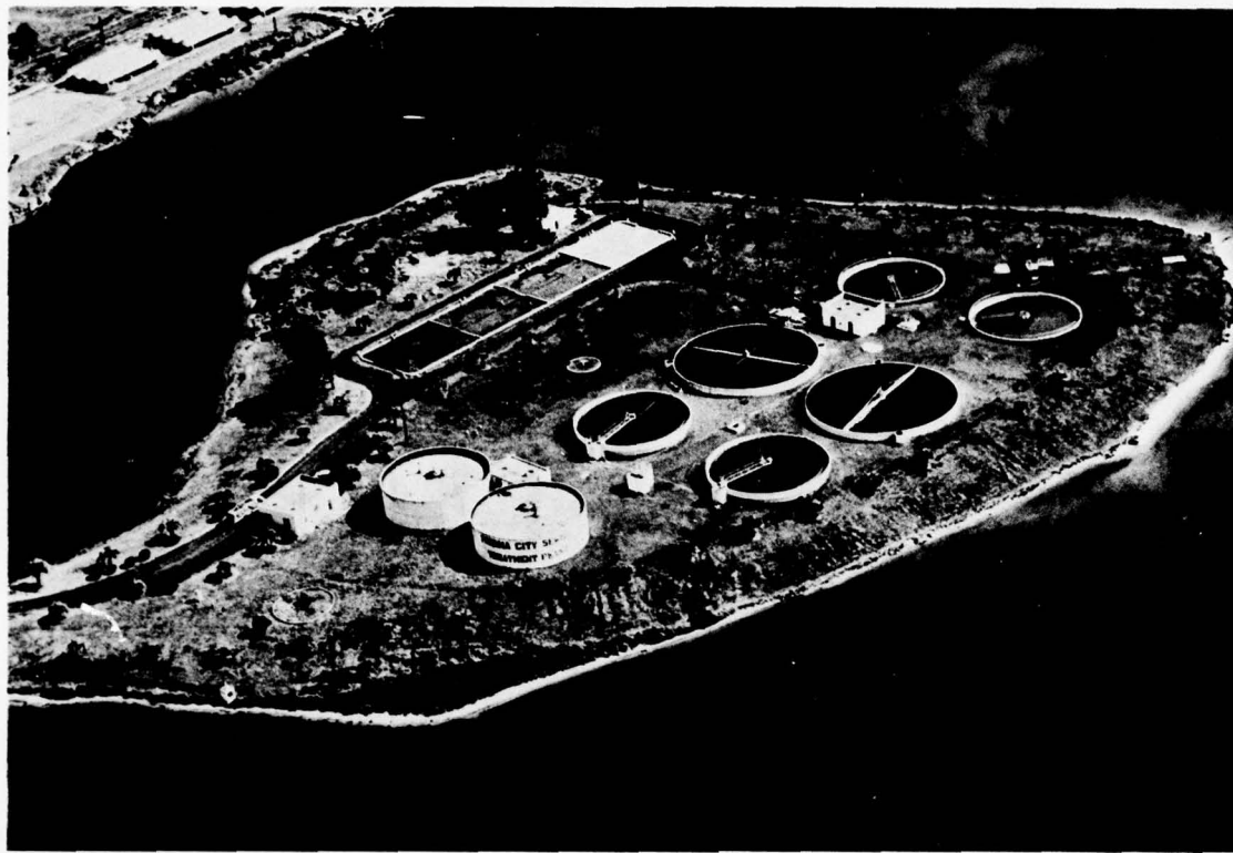
Figure 2.34 Modern Trickling Filter Sewage Treatment Plant.
