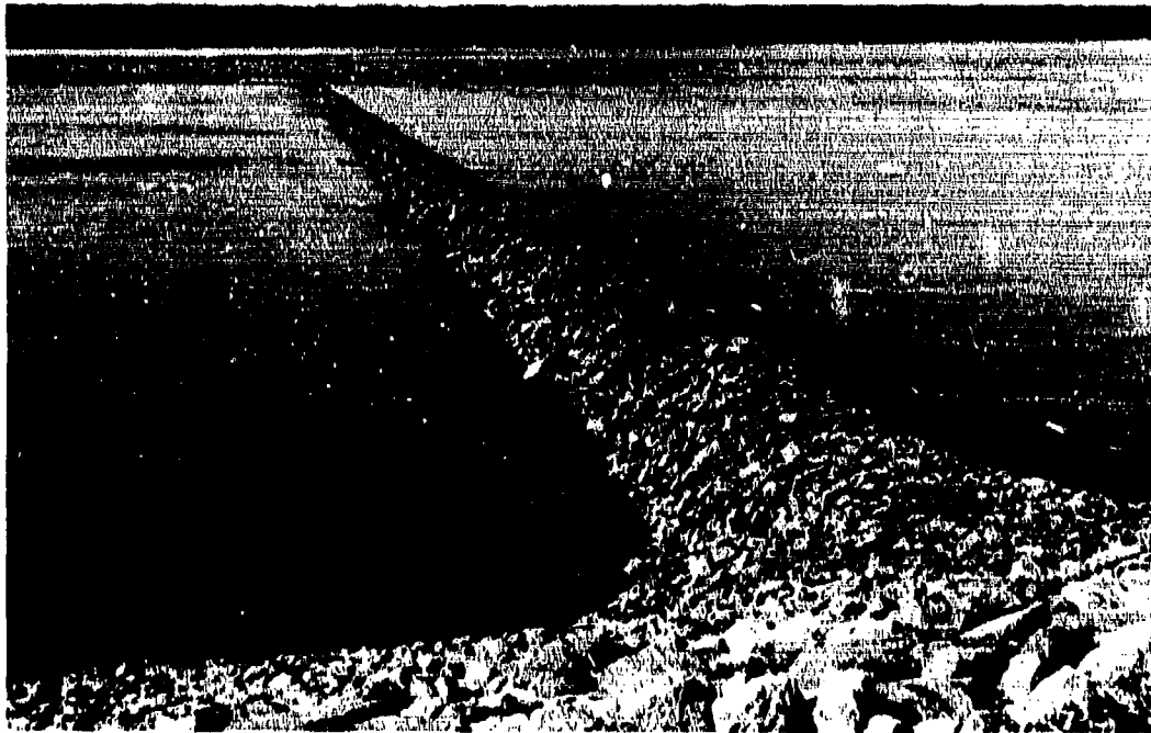
Figure 33. Transverse stone dike
