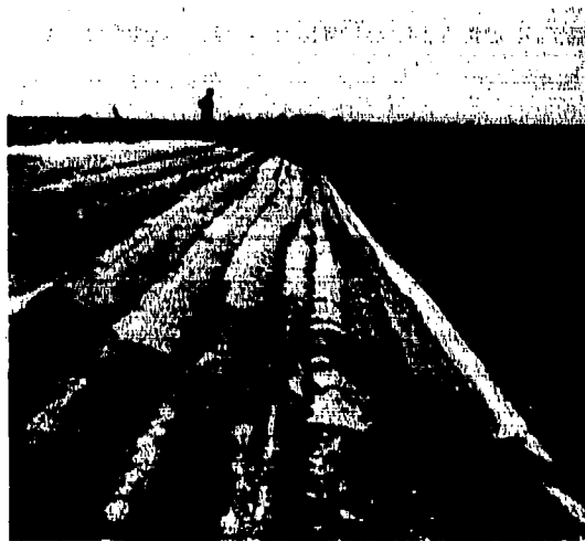
Figure 58. Soil-cement mixture used to pave bank (photo courtesy of Portland Cement Association)
