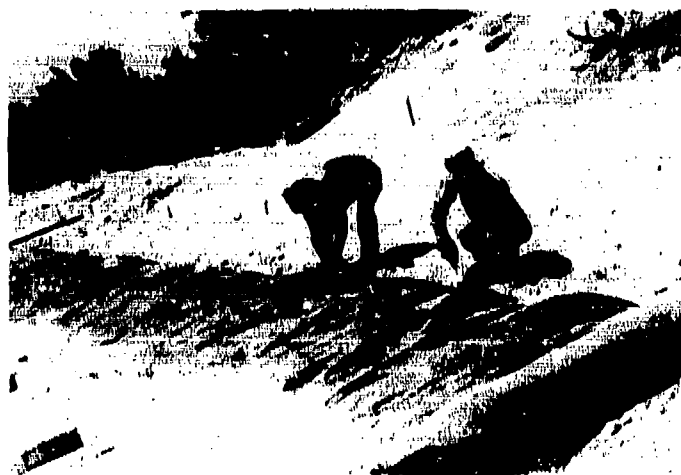
Figure 27. Installation of filter cloth prior to placement of riprap (photo courtesy of the Erosion Control Division, Carthage Mills, Inc.)
