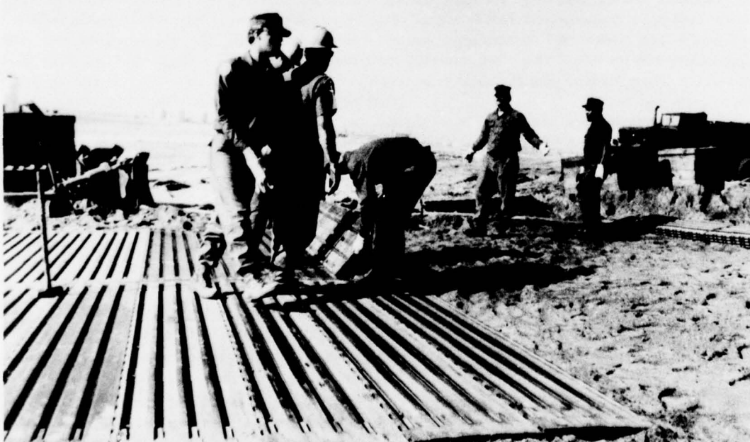
Figure 24. PHIBCB-ONE crew installing M8A1 steel beach matting.
