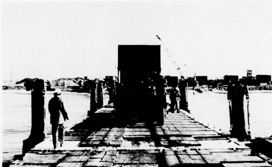
Figure 25. Timber roadway on elevated causeway.
