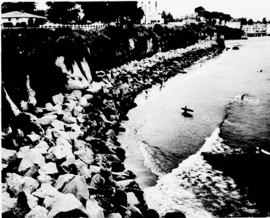
This revetment is a part of the Federal shore-protection work constructed by the Corps of Engineers at Santa Cruz, in the Central Coastal subregion.
