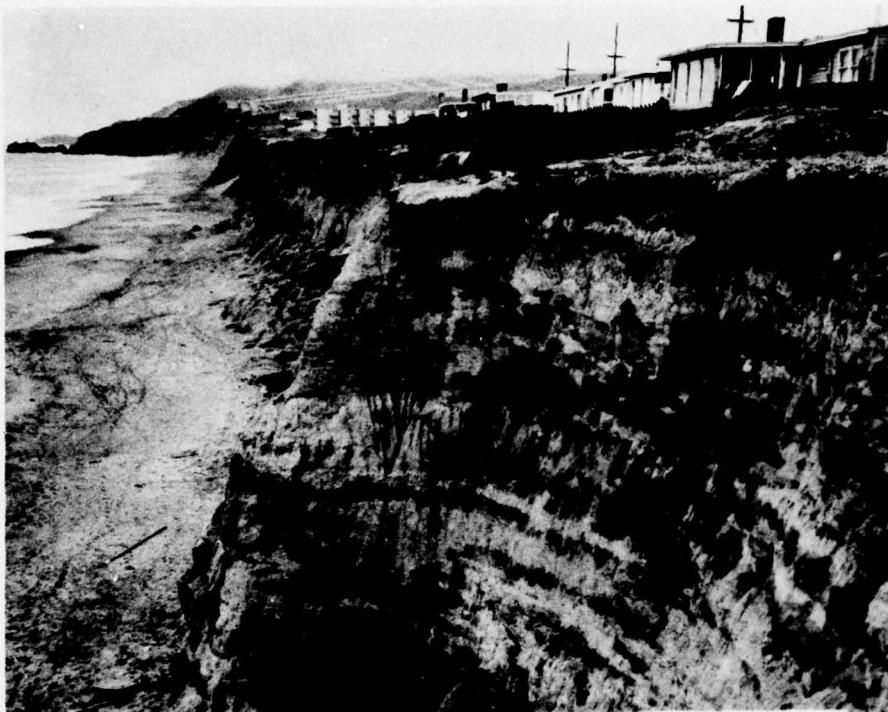
These residences in Pacifica (San Francisco Bay Subregion) are endangered by serious erosion.
