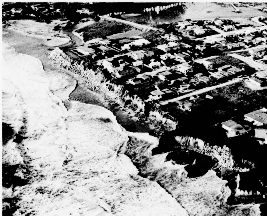
Private property owners have also revetted the shoreline in front of their homes in the Santa Cruz area.
