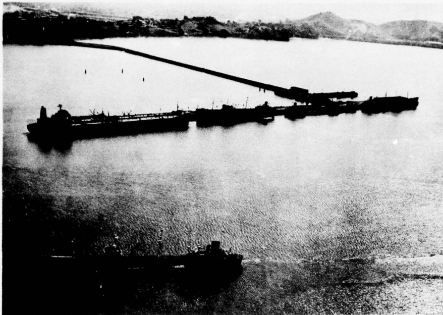
This petroleum terminal in San Francisco Bay will accommodate a supertanker with a draft of 35 feet. The supertanker of the future may have a draft of 70 feet. (Corps of Engineers photo)
