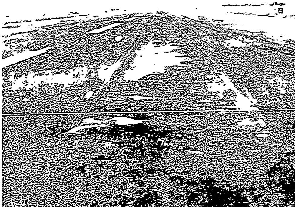
Figure 14. Patched area in porous friction surface.
