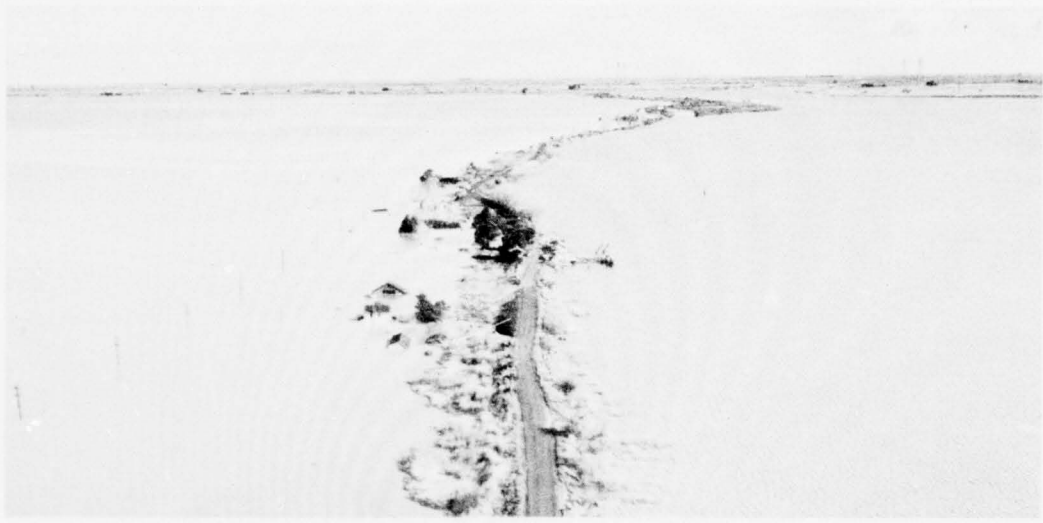
Sherman Island (left of levee road) after levee failure during January 1969. About 10,000 acres were flooded. (Corps of Engineers Photo.)
