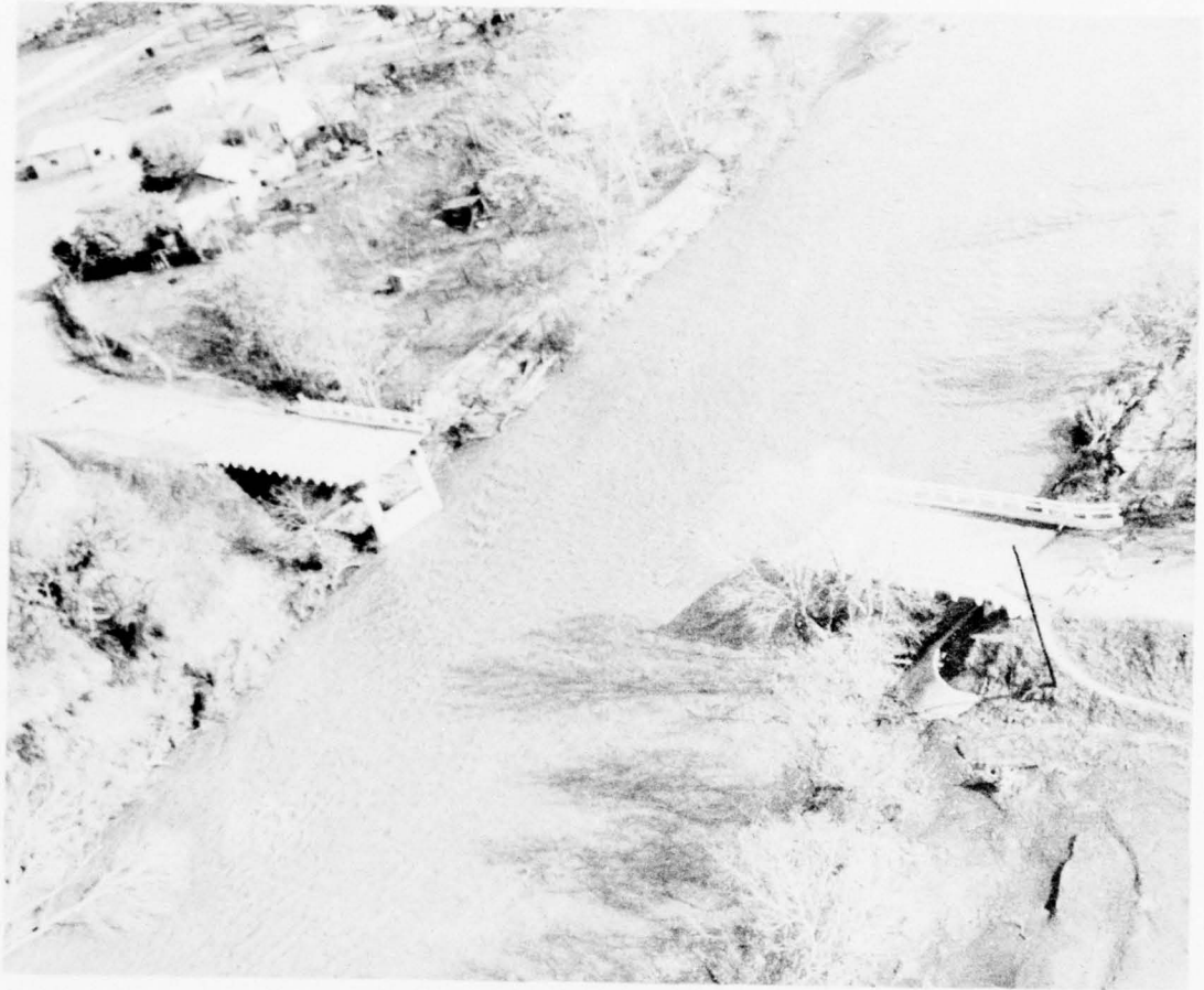
Paskenta Bridge destroyed by record Thomas Creek floodflows, December 1964. (Tehama County Photo.)
