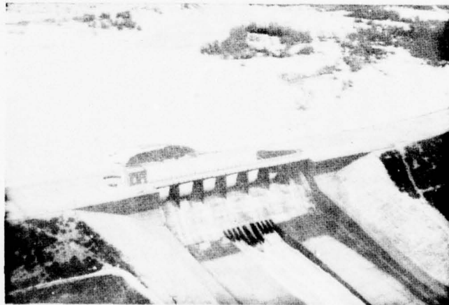
Hansen Flood Control Reservoir on Tujunga Wash, showing discharge during February 1969 flood. (Corps of Engineers Photo.)
