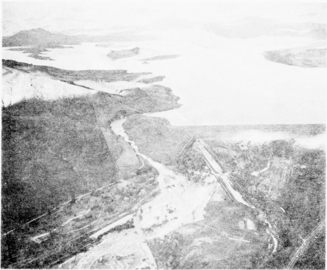
Success Dam and Reservoir on Tule River during the December 1966 flood. (United Aerial Survey Photo.)
