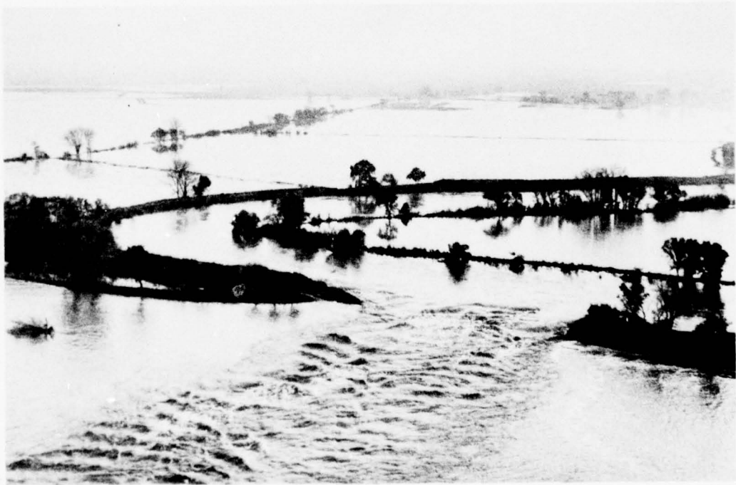
Break in the east levee of San Joaquin River near Mossdale, 1950 flood. (Corps of Engineers Photo.)
