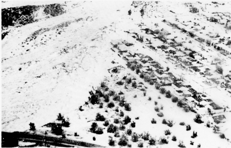
Flood damage along Big Tujunga Wash, Los Angeles, February 1969. (KTLA Telecopter Photo by Harold Morby.)
