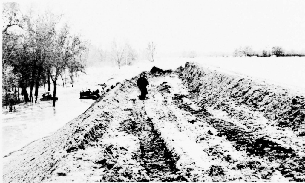
After forty minutes, uncontrolled floodwaters poured through the breached levee to inundate about 25,000 acres of farmland and parts of two nearby towns. Damages were estimated at almost $7 million.
