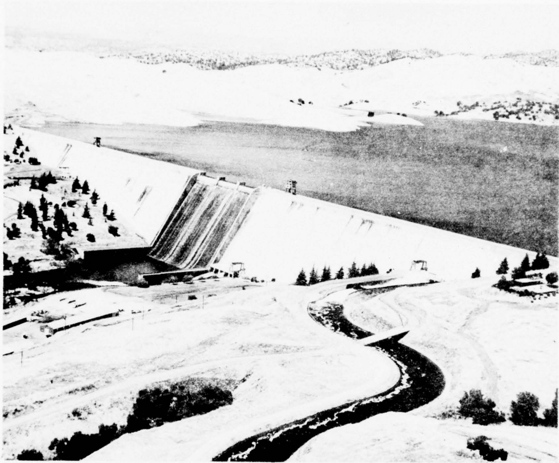
Friant Dam and Millerton Lake on San Joaquin River. A portion of the Friant-Kern Canal appears in the right foreground. (Bureau of Reclamation Photo.)
