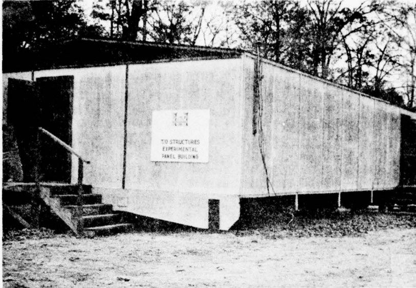
Figure 24. Foam/wood panelized building at USAES after year in service.
