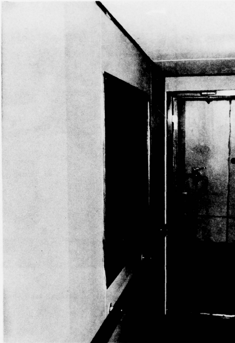
Figure 14: The Lobby, port side of the Diesel Generator Room Casing, No. 01 Deck looking towards the Executive Officer's Washroom.
