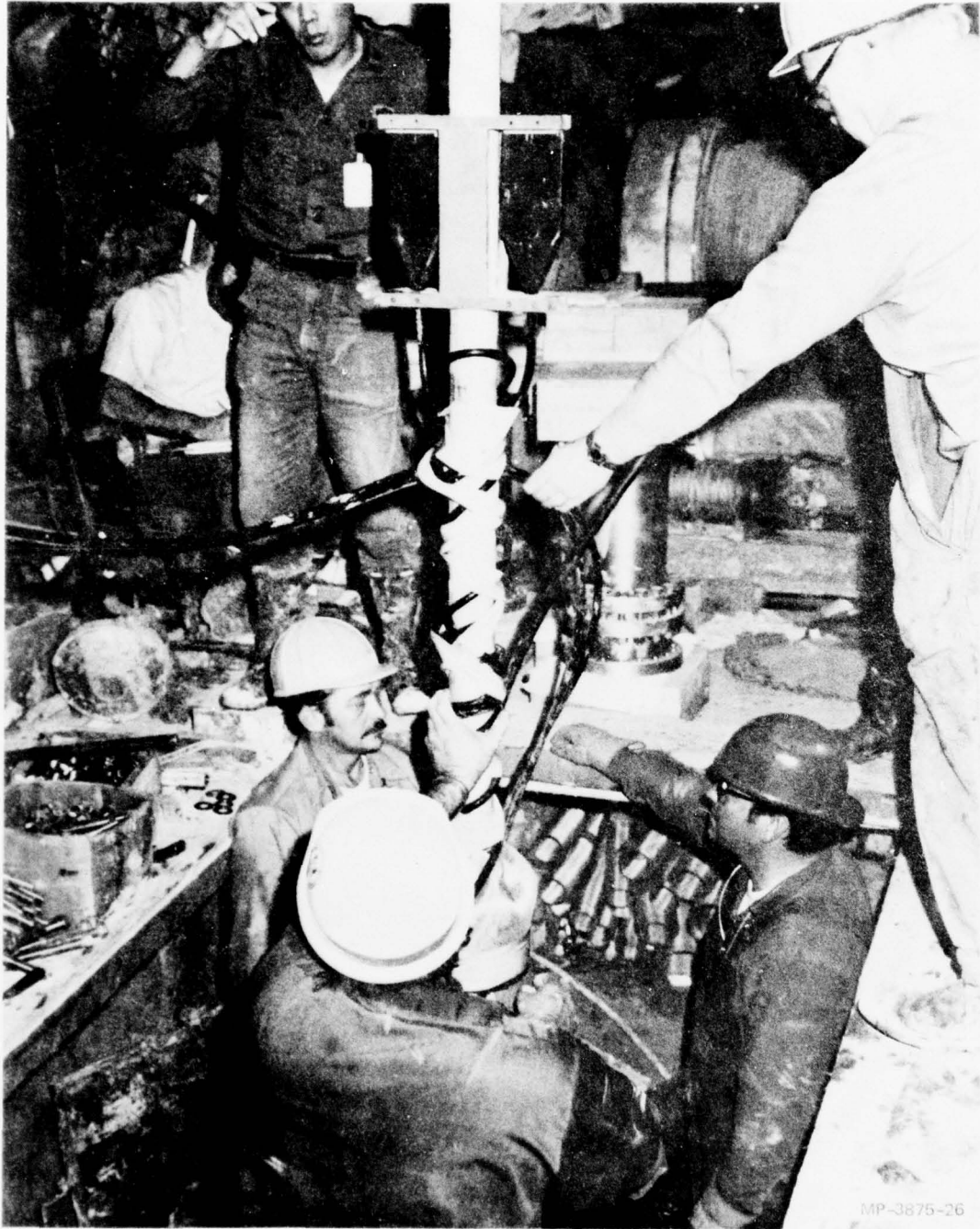
FIGURE 6 GAGES AND HOLDER MOUNTED ON CANISTER CONNECTING TUBE (Courtesy of Waterways Experiment Station)
