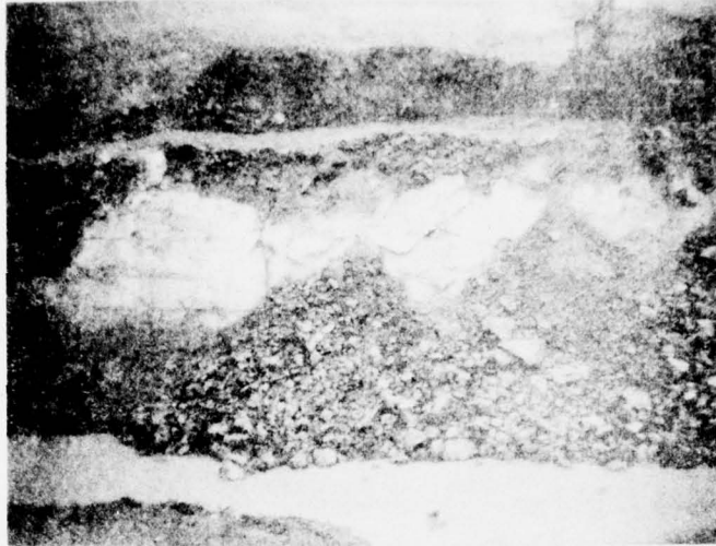
Figure 5. View of central portion of excavation in the diversion channel looking toward the Savannah River showing the smooth, slick pressure faces trending in the dip direction of the fault zone. Apex of the talus cone (left) is at station 18+50. The white, altered felsite zone appearing on the cliff face strikes N 10° E and dips 45° NW.
