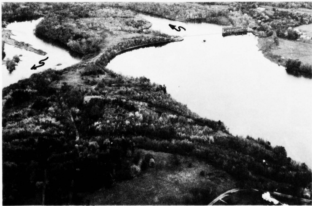
FIG. L-6 VERNON DAM AND POTENTIAL LOCK SITE ACROSS NARROW NECK OF LAND AT EAST SIDE OF THE RESERVOIR
