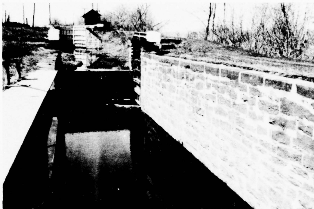
FIG. L-1 PRESERVATION OF LOWER LOCKS TO WINDSOR LOCKS CANAL FOR CONSIDERATION BY LOCAL INTERESTS
