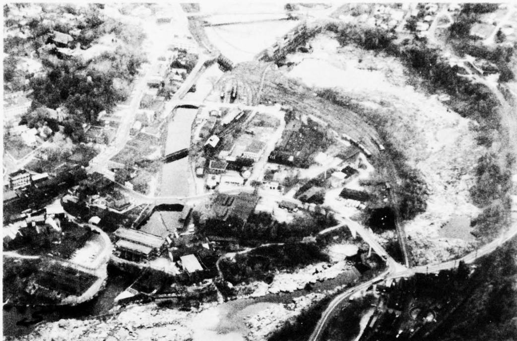
FIG. L-7 BELLOWS FALLS DAM, POWER CANAL, AND CONGESTION OF RAILROADS, BRIDGES, AND BUILDINGS
