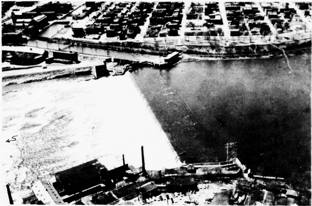
FIG. L-3 HOLYOKE DAM AND REMNANTS OF WILLIMANSETT CANAL IN FOREGROUND
