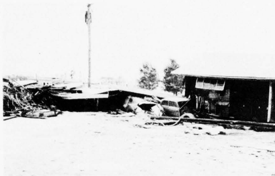
Damage to cars and a duplex in Denver, Colorado, from the 1965 South Platte River flood.
