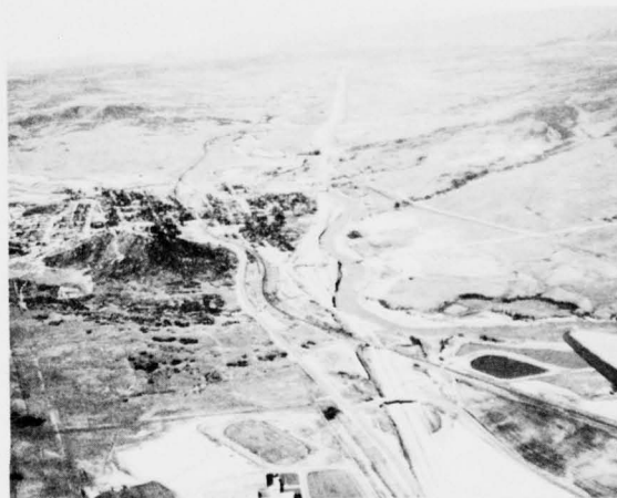
Streambank erosion along an interstate highway near Castle Rock, Colorado.
