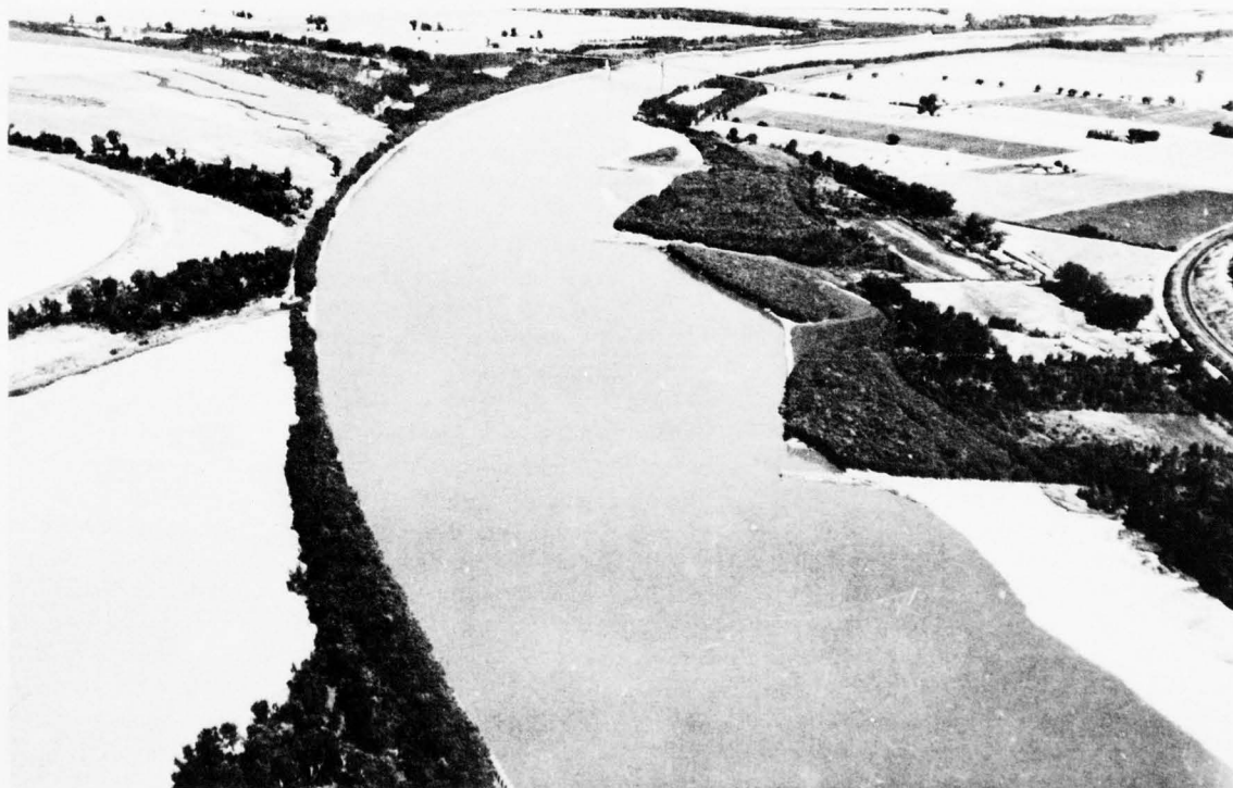
Integrated bank stabilization works and reservoir operation overcome bank erosion and regulate flows permitting navigation.
