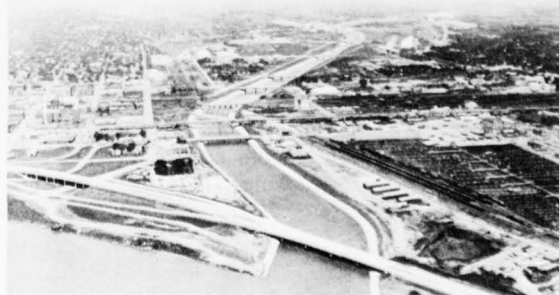
Completed Floyd River channel improvement project at Sioux City, Iowa.
