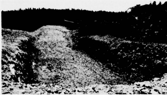
Fig. 3. Completed cut. View toward the south
