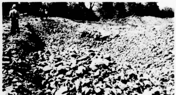
Fig. 6. Rubble from second-lift blast fills first-lift trough. Presplit surface at left
