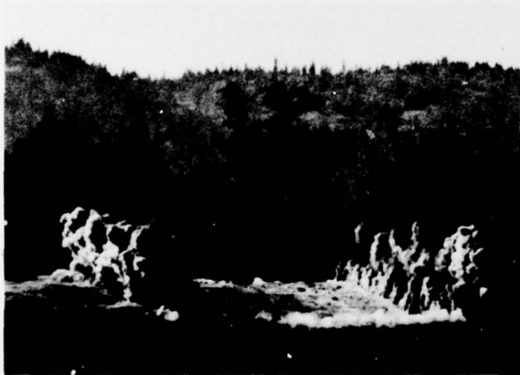
Fig. 4. First-lift detonation, showing presplit and buffer zones already detonated with mounding charges to follow shortly
