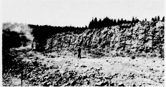
Fig. 5. First lift fully excavated. Plywood squares cover second-lift charge emplacement holes
