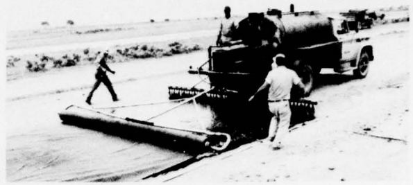
Fig. 4. Installing upper membrane
