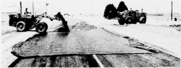
Fig. 3. Placing soil on lower membrane
