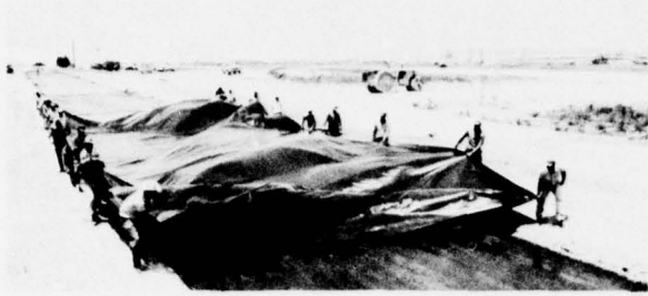
Fig. 2. Installing lower membrane
