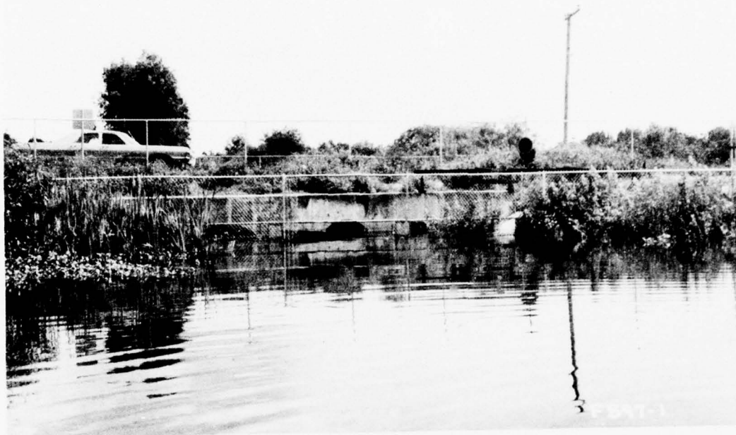
Figure 3. Culverts (structure 1) under Daetwyler Drive
