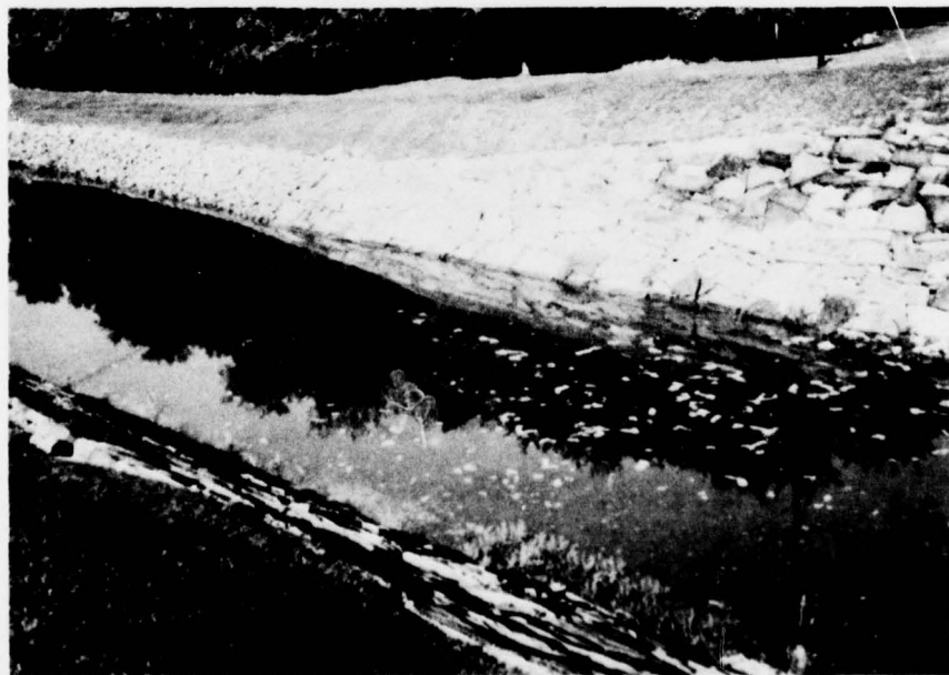
Photograph 4. Clendening Lake, view downstream of stilling basin
