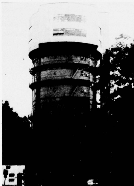
Figure 1. External View Undersea Weapons Tank.
