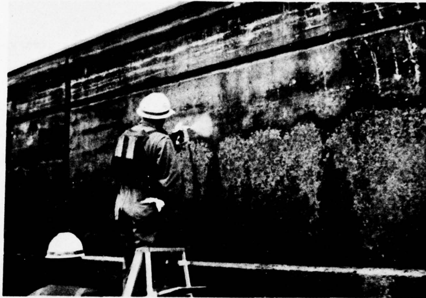
Fig. 3. Applying coating to the lock wall
