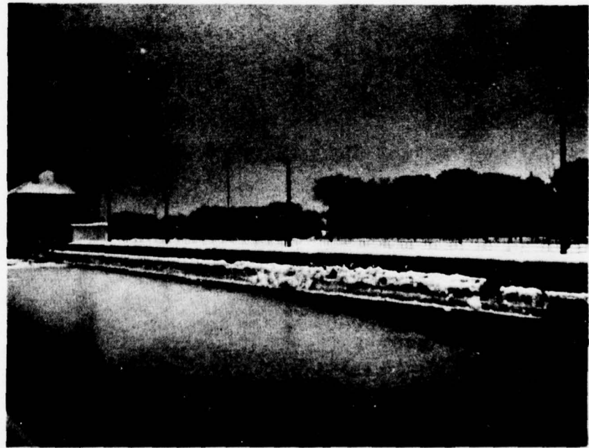
Figure 3. Deep ice collars at Poe Lock.
