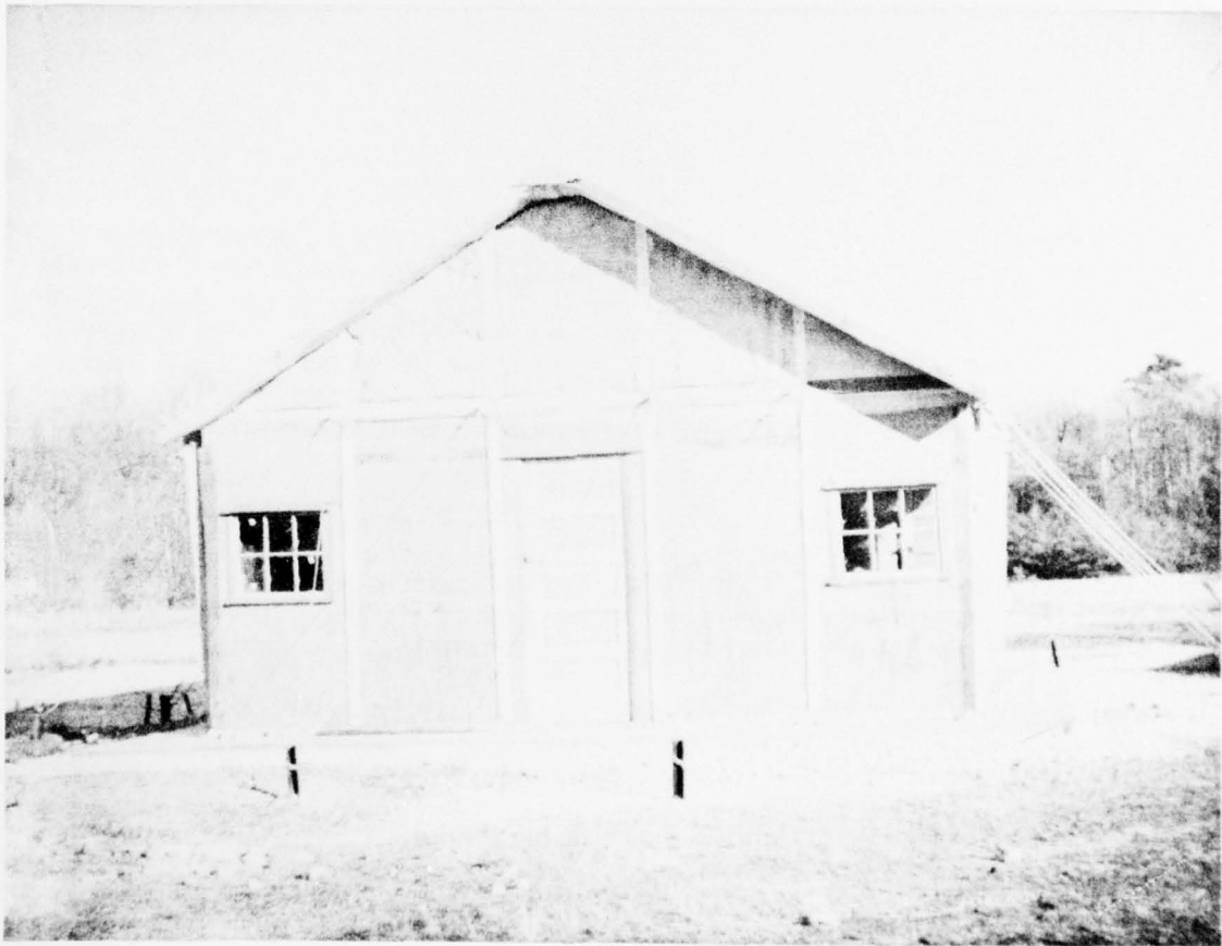
Figure 3. Completed foam building at USAES.
