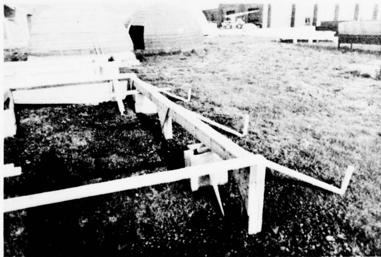
Figure 11. Completed laminated-girder foundation system.
