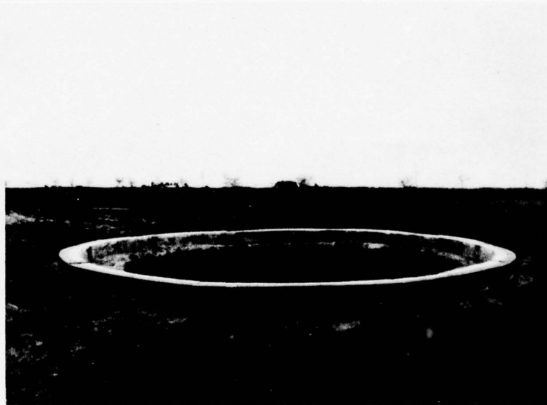
Figure 8. Ring beam for 28-ft (8.5-m) diameter dome.
