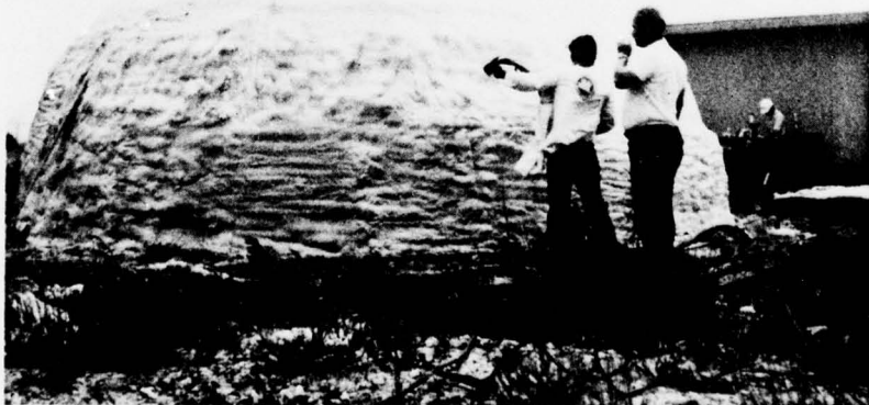
Figure 14. Foam application on 28-ft (8.5-m) diameter dome.
