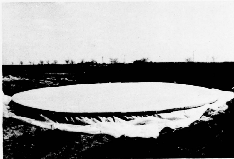
Figure 9. Bottom membrane for 28-ft (8.5-m) diameter dome.
