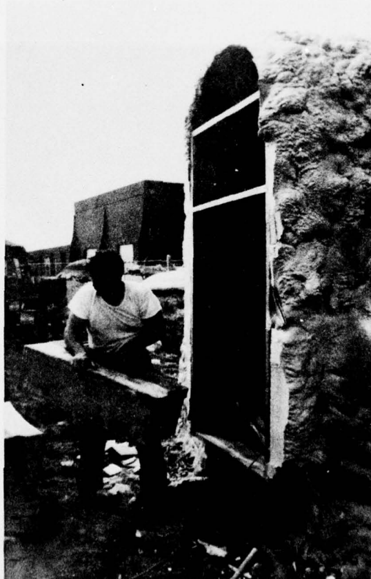
Figure 18. Removal of wedge-shaped key ring beam section.
