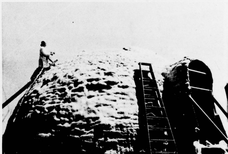
Figure 15. Ladder used in foaming operation.
