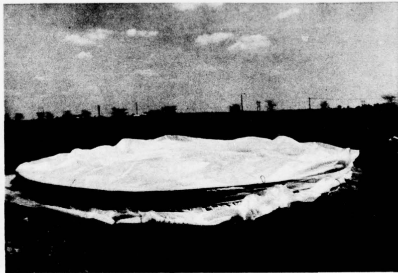
Figure 10. Top membrane for 28-ft (8.5-m) diameter dome.
