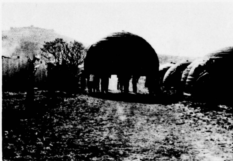
Figure 4. Short distance transport of completed dome.
