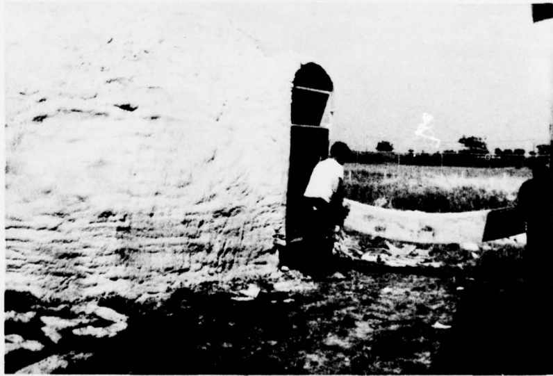
Figure 20. Removal of ring beam sections.
