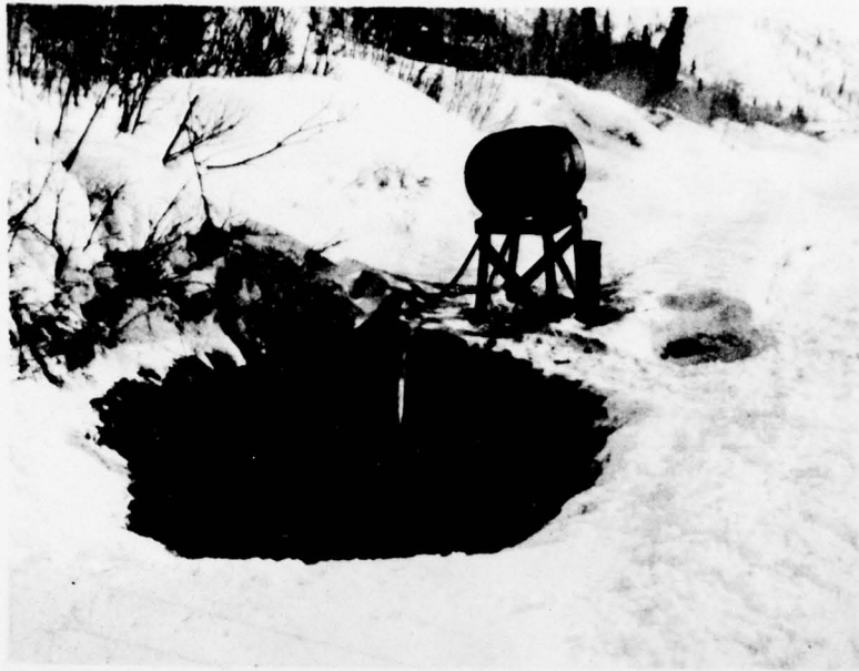
Figure 7. A typical firepot installation at the entrance to a culvert. The firepot has created a thaw pit in the ice. The culvert entrance is out of sight in the thaw pit, and the fuel supply is beyond the thaw pit.
