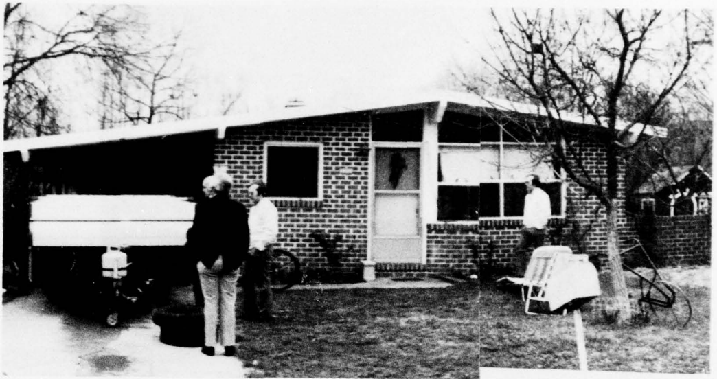
Slab-On-Grade: 1700 Sunny Court Drive Baltimore, MD
