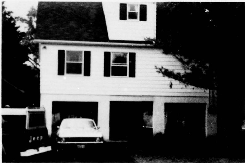
House Raising - Leaving Basement Area Open Lock Haven, PA
