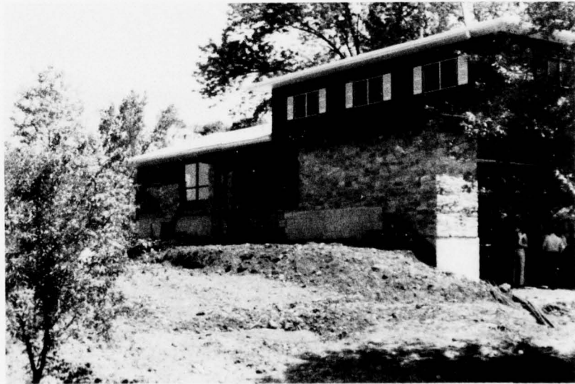
House Raising With New Block Foundation Harrisburg, PA
