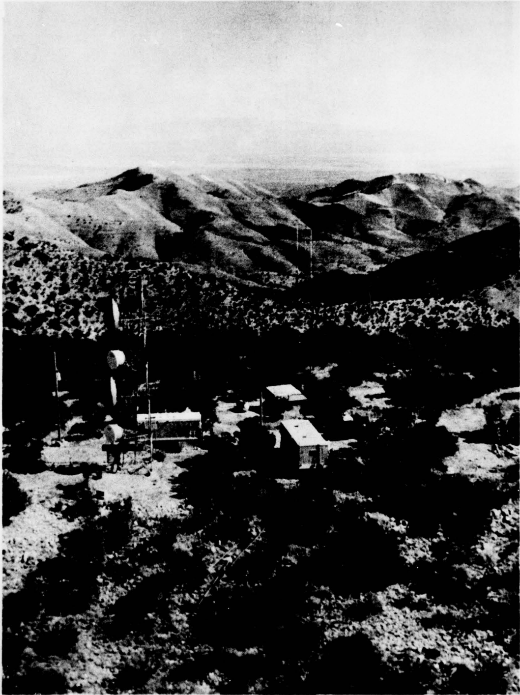
Figure 3. Photograph of Mule Mountain Microwave Site
