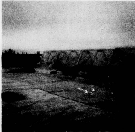
Figure 6. The A-frame shelter is placed over a lap joint to be made.
