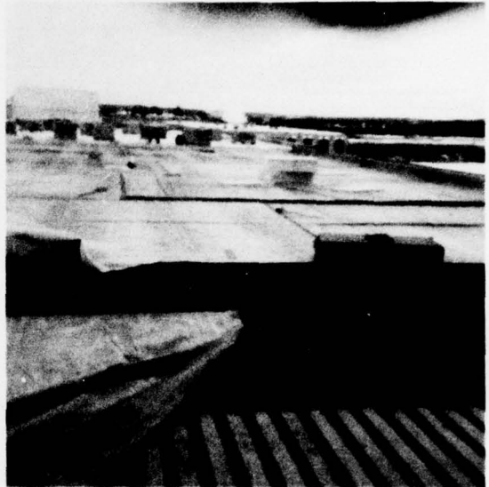
Figure 3. Metal deck, underlayment and sheet rubber membrane during roof installation.
