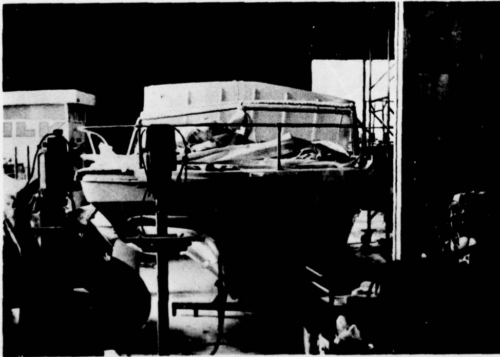
FIGURE 6. DAMAGE TO BOAT NO. 1
