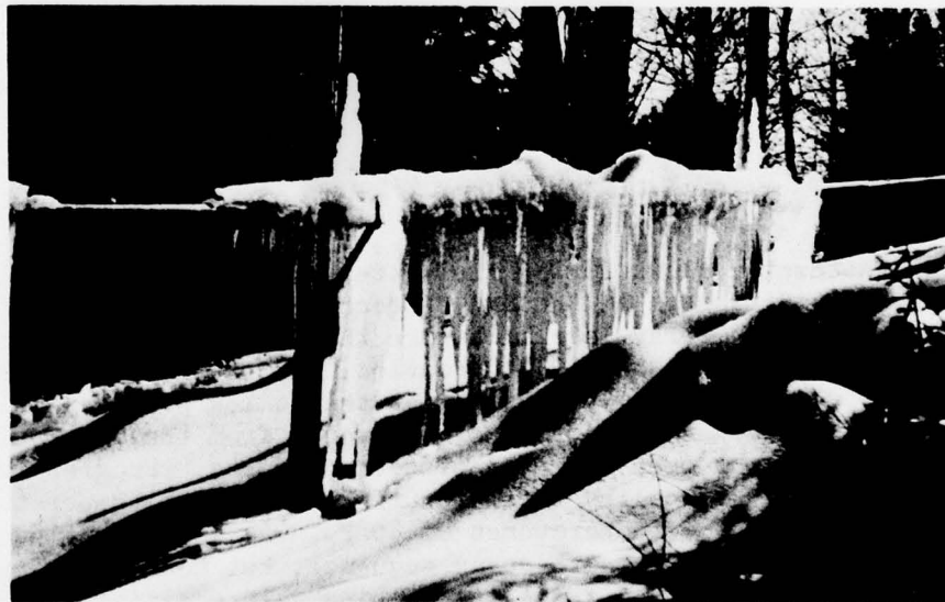
Figure 5. Ice buildup on spray laterals.
