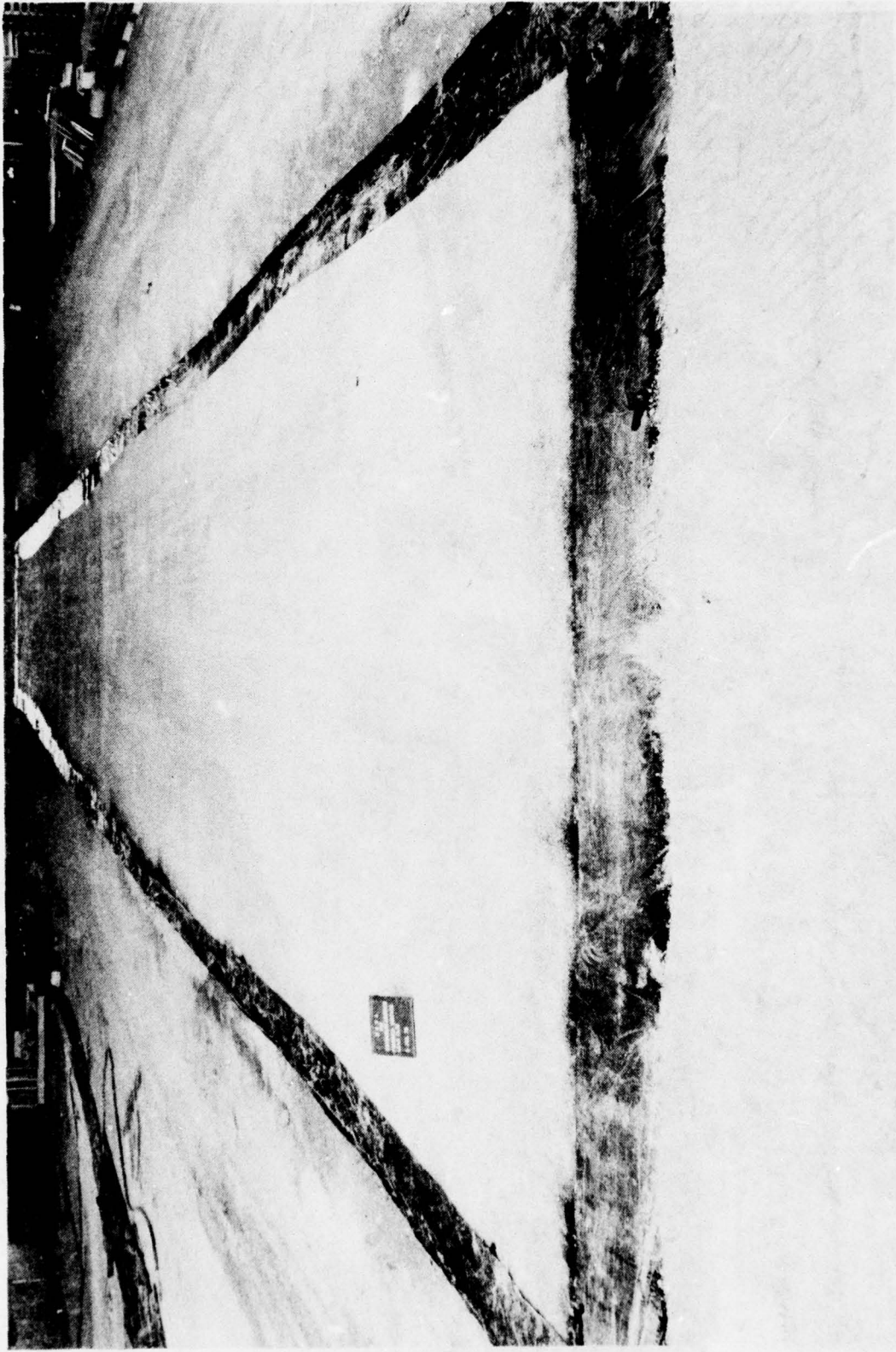
Figure 17. Finished Surface of Lean Clay with Polyethylene Folded Over Edges
