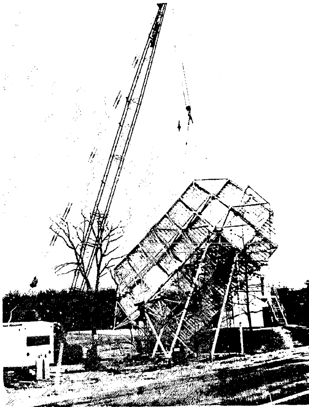
Figure 6-21. View of COMSAT UET Torus Antenna During Construction
