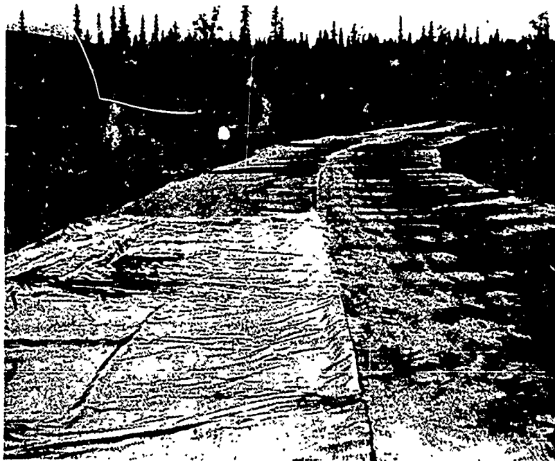
Figure A7. Subgrade membranes in place with lapped joint sealed.
