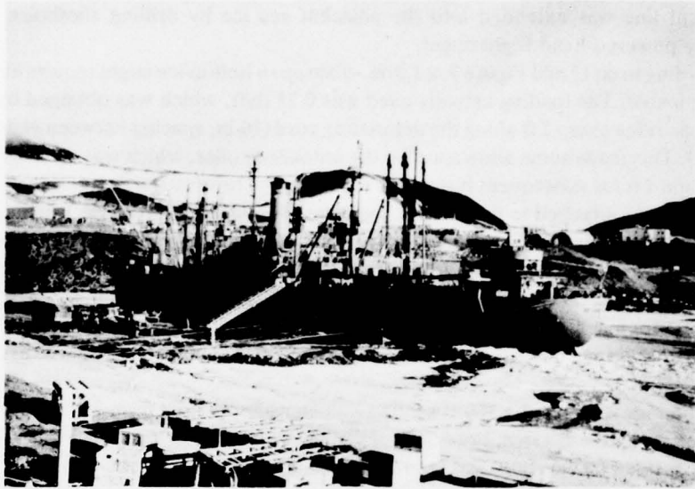
Figure A2. USNS Pvt. John R. Towle tied up against the trimmed face of the McMurdo ice wharf after the blasting operation of January 1975.
