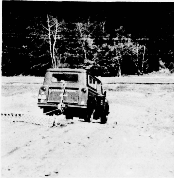
Figure 18. Dragging slope with wire fence loaded with concrete block.
