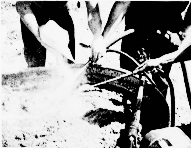
Figure 20. Mixing Terra Tack II into the wood fiber mulch using high pressure water streams.
