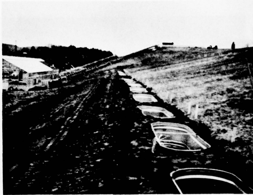
Figure 8. Final grade. Note small berm on lower slope to retard erosion during construction.
