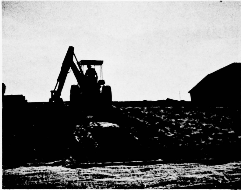
Figure 10. De-sodding test plot with backhoe.
