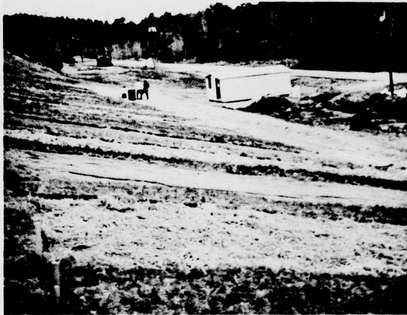
Figure 13. Completed sediment tank test plots.
