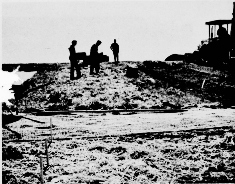
Figure 12. Four test plots in various stages of completion.
