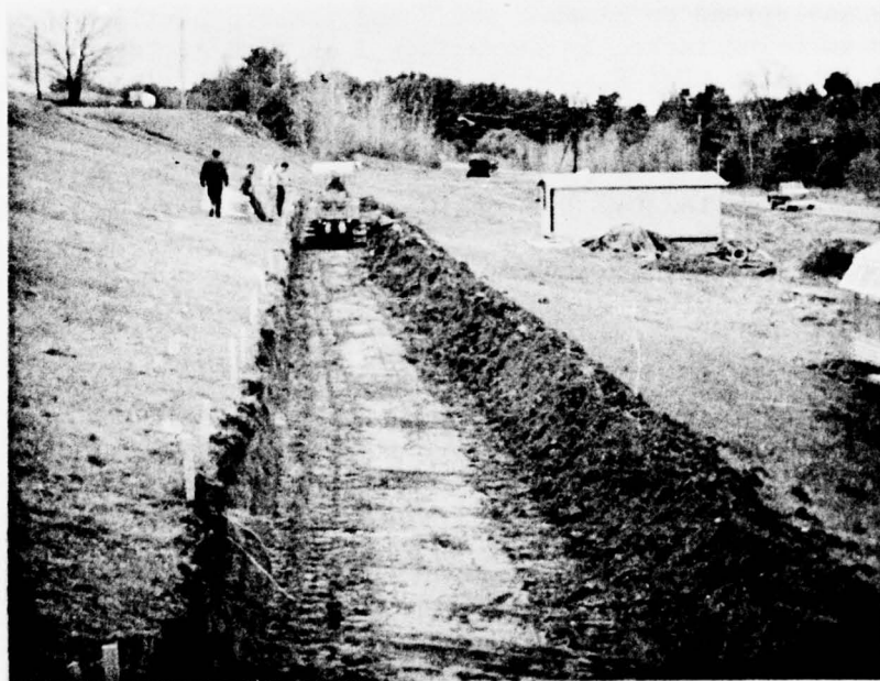
Figure 3. Initial cut for placement of the sediment tanks.
