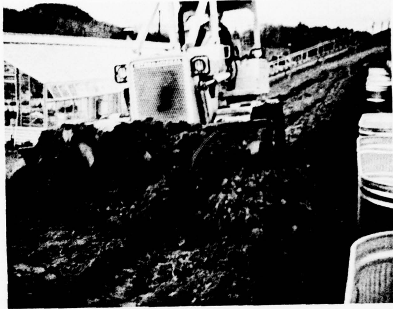
Figure 6. Backfilling the area around the sediment tanks.
