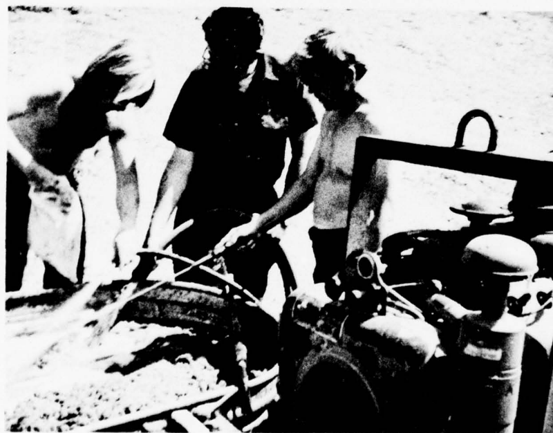
Figure 21. Pump used to mix Terra Tack II and wood fiber mulch.
