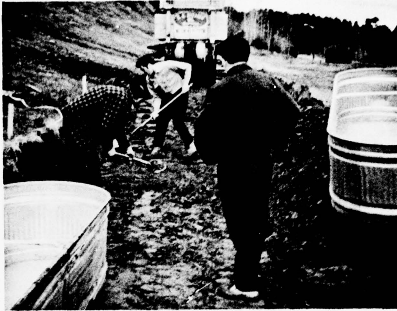
Figure 4. Hand leveling of the area just prior to placement of the sediment tank.
