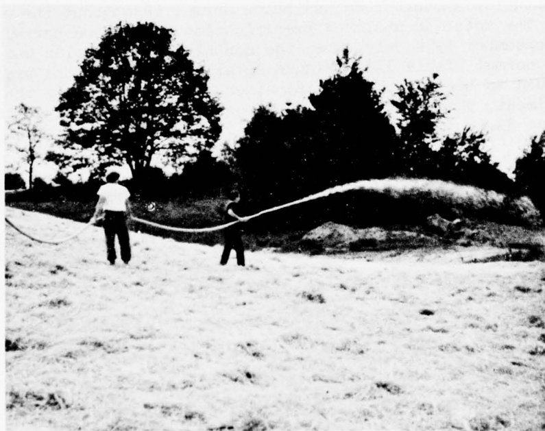
Figure 25. Spraying Dow latex chemical on straw.
