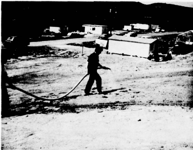
Figure 23. Spraying Terra Tack II directly on soil.
