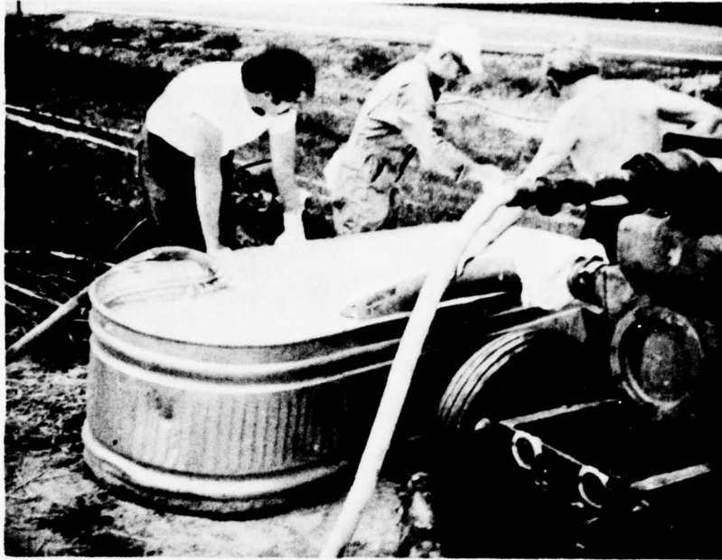
Figure 22. Mixing Dow latex chemical just prior to application.
