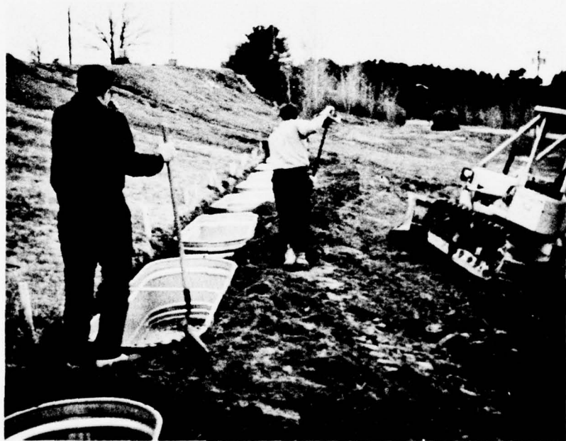
Figure 7. Soil being pushed up to the tanks for final grade.
