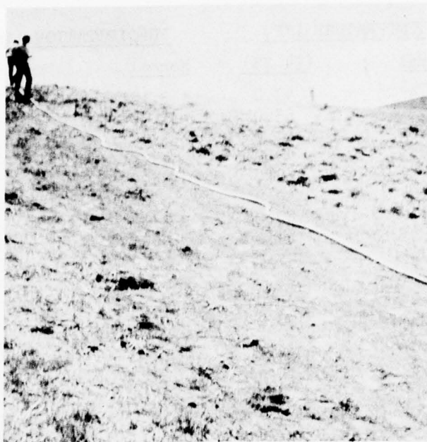
Figure 24. Tacking straw with Terra Tack II.
