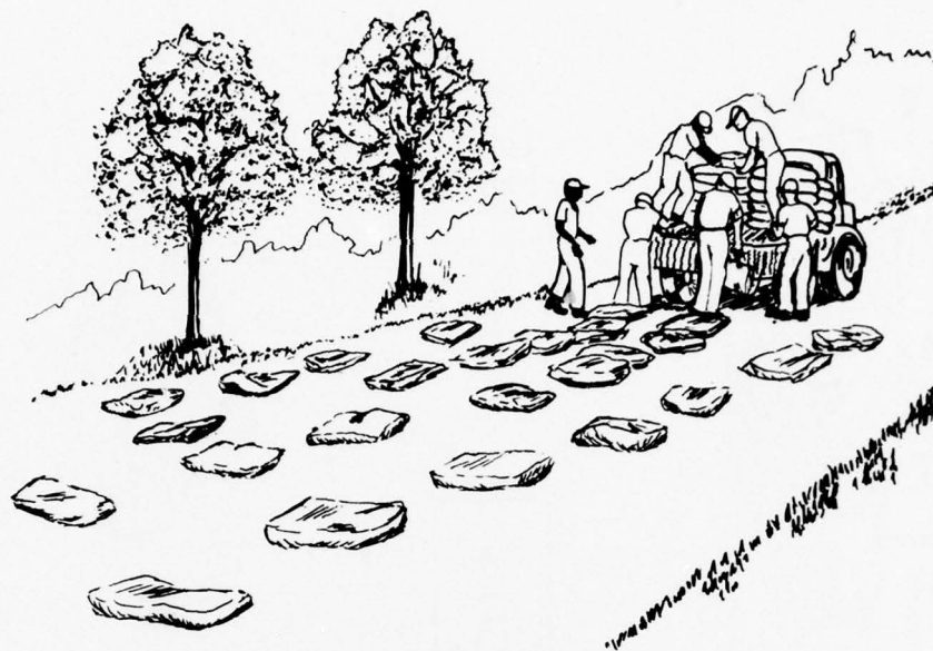
Figure 10. Spreading the stabilizer
