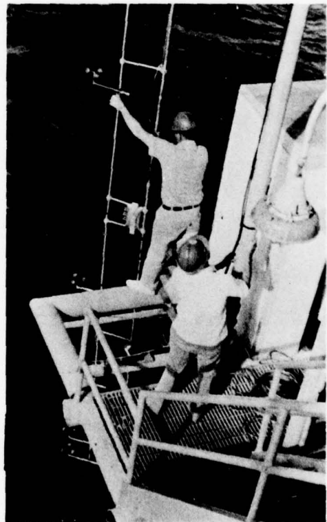
Figure 12. A photograph of the Thornthwaite Wind Profile Register System on an offshore platform (PG-3, Petrobras). Note that the working catwalk is about 14 meters above the mean water surface.
