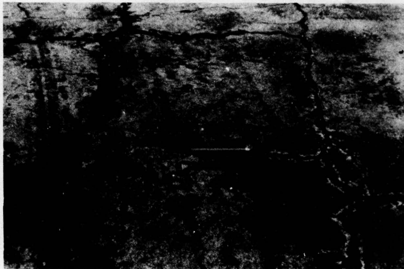
Figure 17. Medium Severity Block Cracking.
