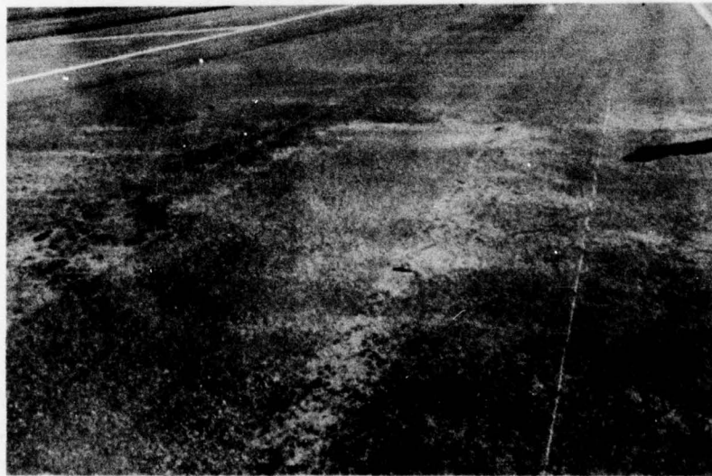
Figure 23. Medium Severity Corrugation.
