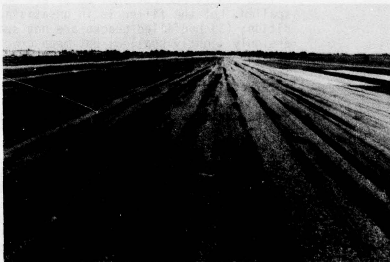
Figure 39. Low Severity Longitudinal Cracks, Approaching Medium.
