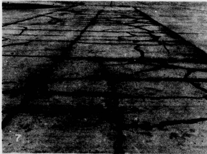
Figure 124. Shattered Slab.
