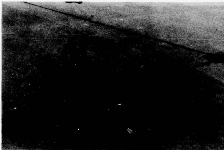
Figure 81. Low Severity Diagonal Crack.
