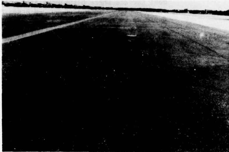
Figure 27. Medium Severity Depression (> 1/2 Inch).
