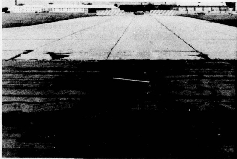
Figure 70. High Severity Sharp Swell.
