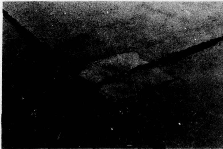
Figure 96. Low Severity Small Patch.
