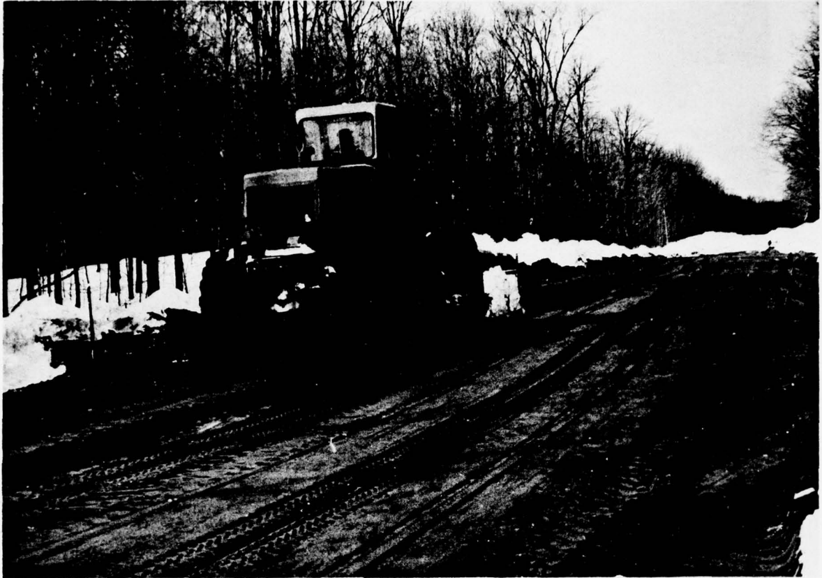
7. Ontonagon County. North Firesteel Road. Back blading and final compaction at end of the working day. Low overnight temperatures freeze fill, creating stable roadway by the next morning.
