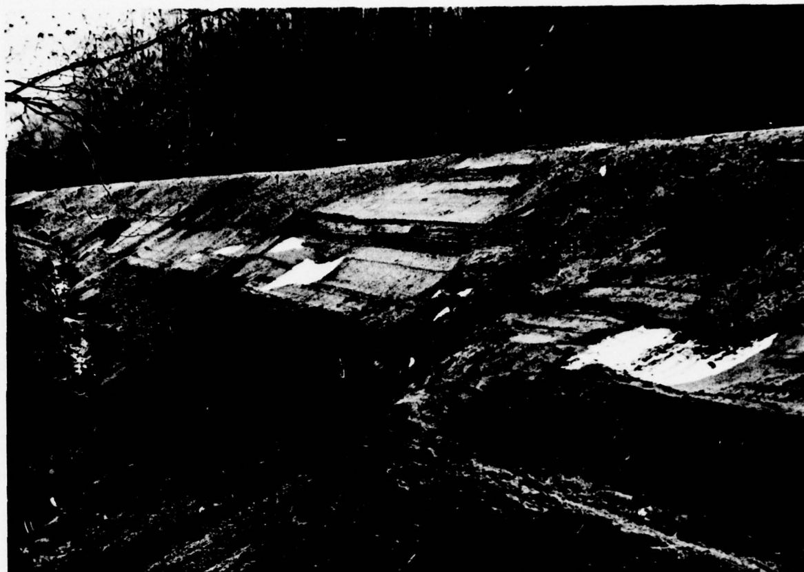
14. Ontonagon County. North Firesteel Road. Evidence that chunks of snow were inadvertently incorporated into slope of fill. Photo taken after slope finishing operation.
