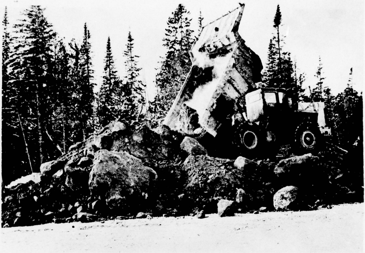
25. Alger County. State Road 28. Placing bouldery clayey soil in zone outside of structural core. Although this soil is not frozen, it was excavated, hauled and placed during the winter, and illustrates how frozen soil could be handled and utilized if necessary.
