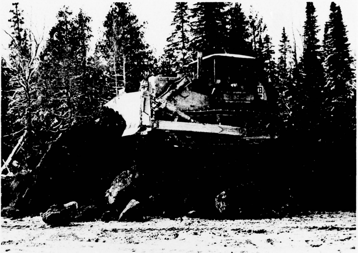
26. Alger County. State Road 28. Spreading bouldery clayey soil (see also Photo 25). Although this soil was not frozen during excavation and placement, the boulders can be considered to act like frozen soil chunks in the fill. Possibilities exist for the formation of large void spaces in the fill.
