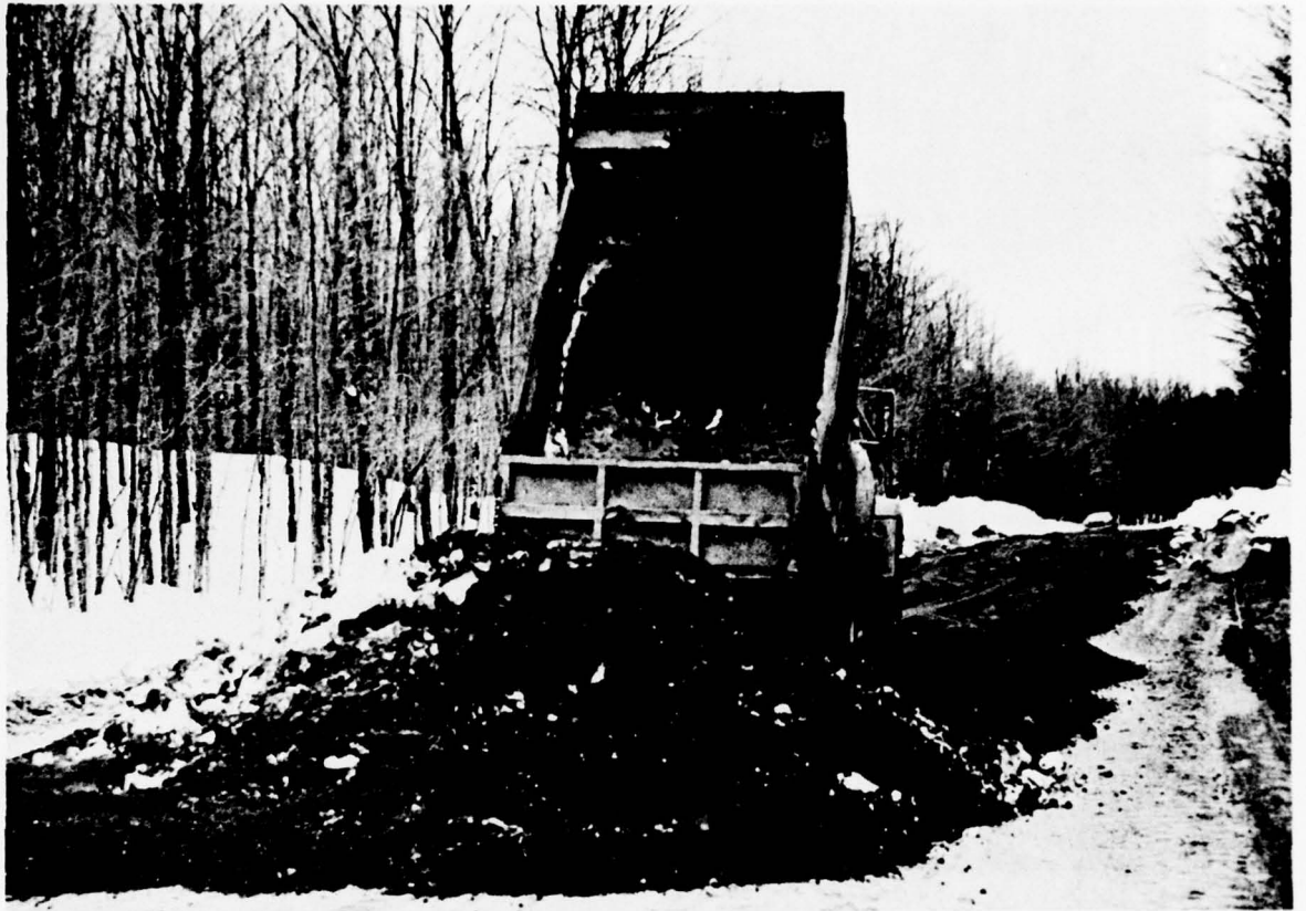
8. Ontonagon County. North Firesteel Road. Sand fill will not bear traffic upon thawing, so gravel surfacing is placed before thawing begins. Gravel is hauled from stockpiles built up the previous summer. Note that considerable snow is included with the gravel.
