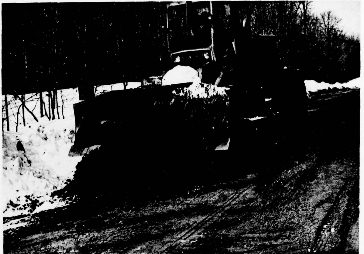
6. Ontonagon County. North Firesteel Road. Another view of spreading and compaction of fill.
