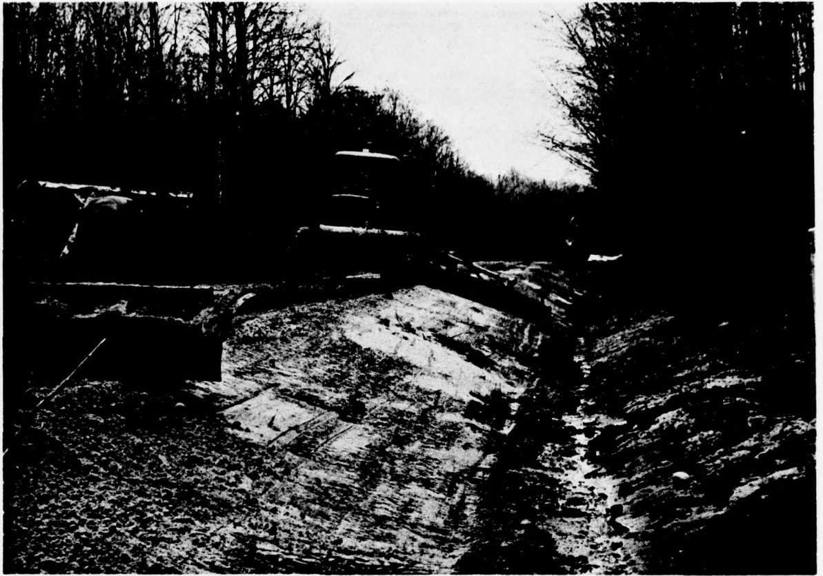
12. Ontonagon County. North Firesteel Road. Another view of slope finishing grader team. Shaping is considered complete after two passes of team.
