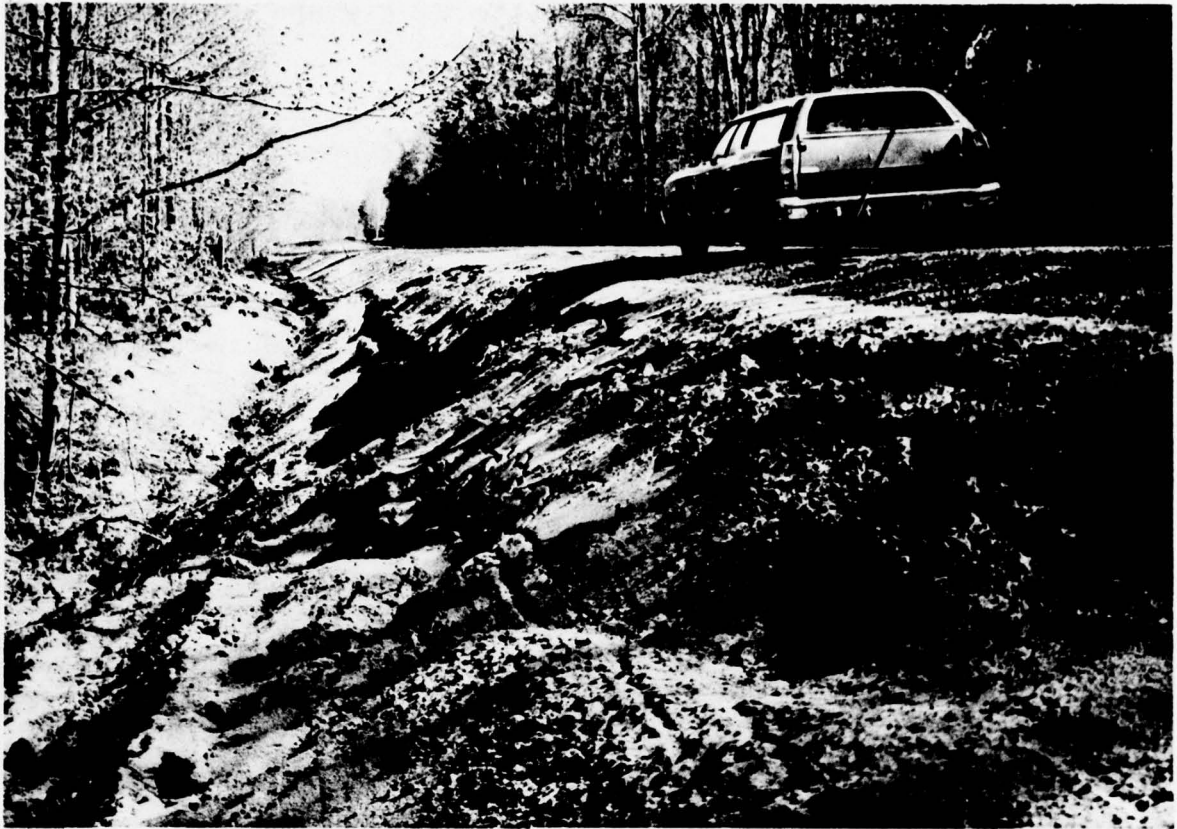
15. Ontonagon County. North Firesteel Road. Slumping of slope, probably due to thawing of frozen soil or incorporated snow. It should be noted that compaction of this part of the fill is difficult due to the construction methods.
