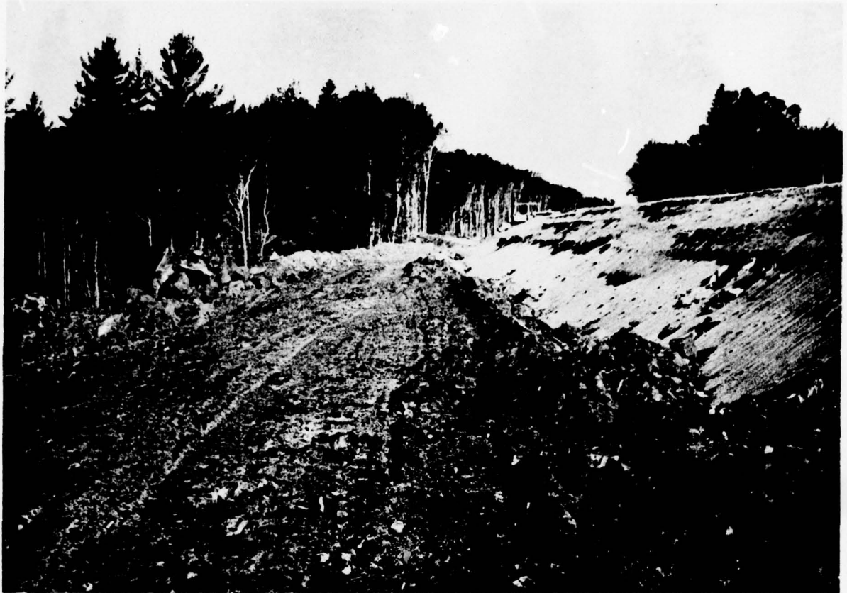
27. Alger County. State Road 28. This photo, taken in summer, illustrates the use of a structural core of sand in the embankment, flanked by less desirable soil in the slope zone. This bouldery clayey soil was placed unfrozen during the winter (see Photos 25 and 26), subsequently froze, and then was compacted and shaped after thawing. Photo taken in June 1976.
