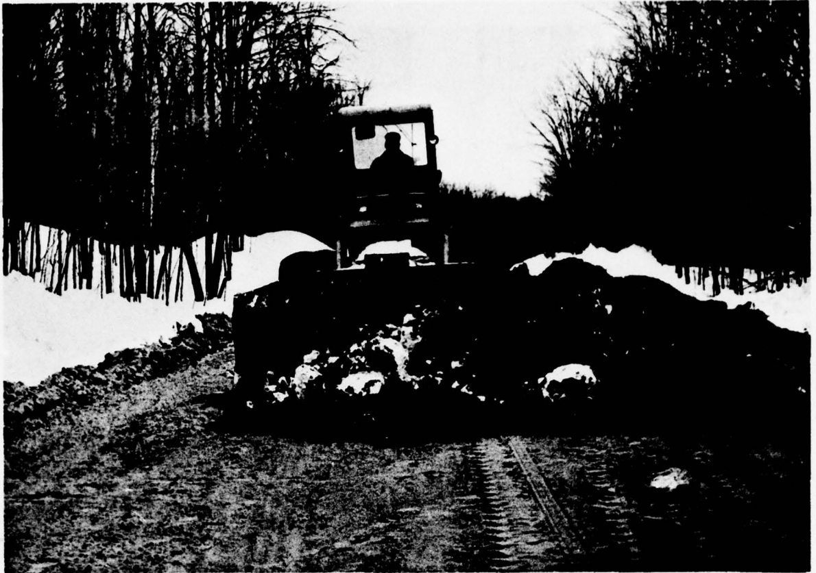
9. Ontonagon County. North Firesteel Road. Spreading and compaction of gravel with rubber-tired dozer.
