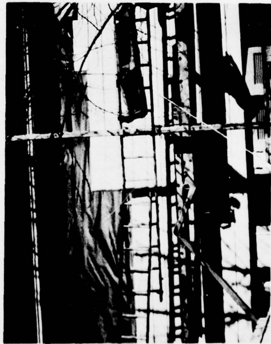
CLOSE-UP OF APARTMENTS DURING INSTALLATION OF ALUMINUM SIDING.
