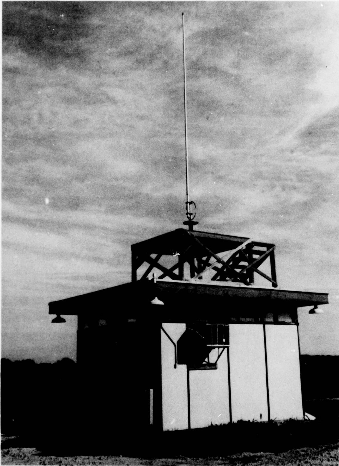
FIGURE 12. TEST SITE WITH COAST GUARD ANTENNAS
