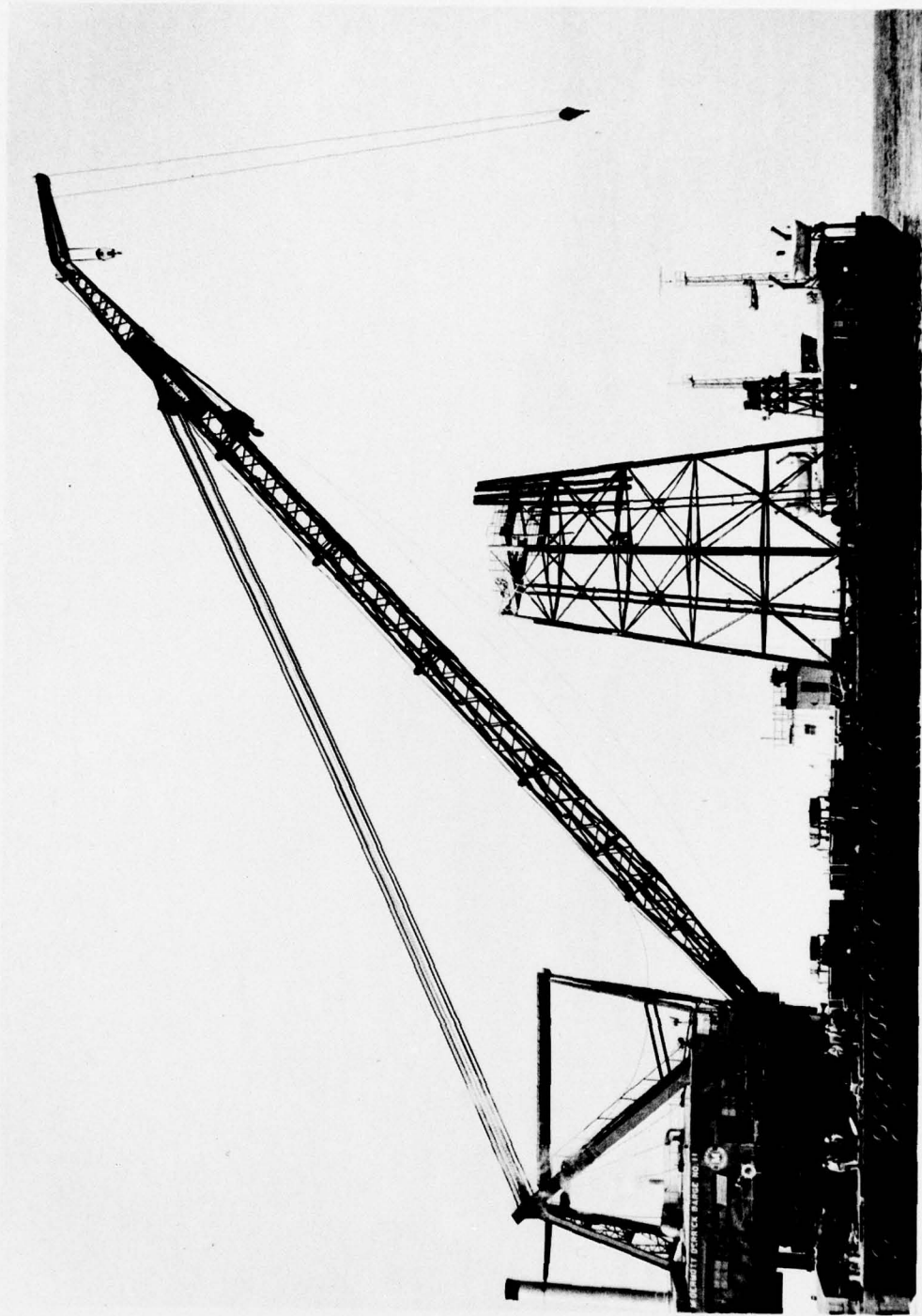
Figure 6. Tower being transported by large barge and crane. (11 June 1959)
