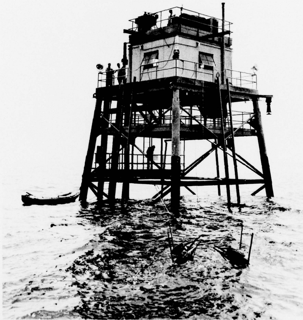
Figure 10. Final tower installation. (24 June 1959)
